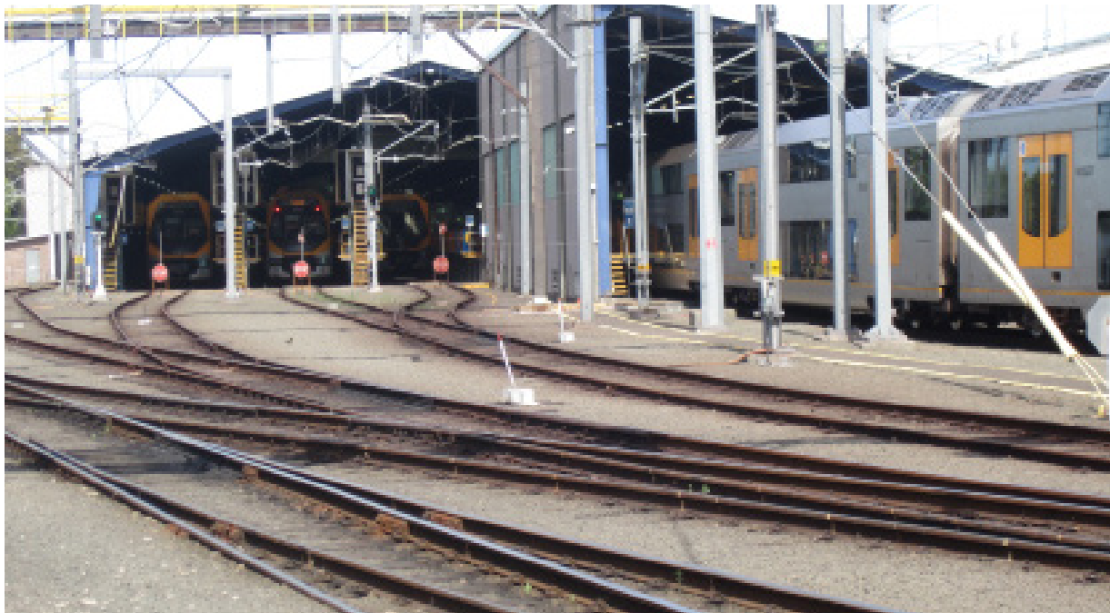
The existing Eveleigh Maintenance Facility.
