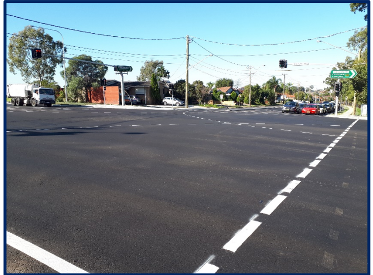
New turning lanes on Merrylands Road (facing eastwards)
