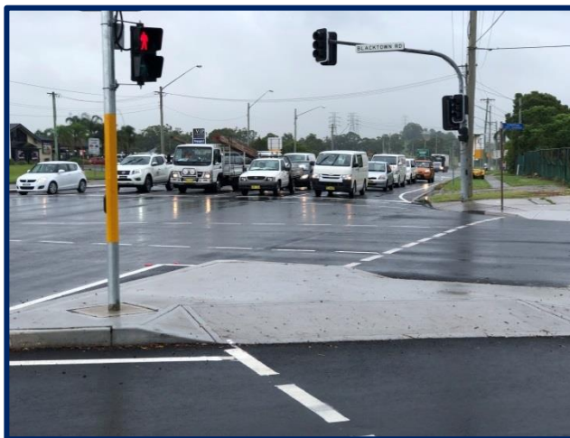
Blacktown Road in Prospect: New pedestrian island
