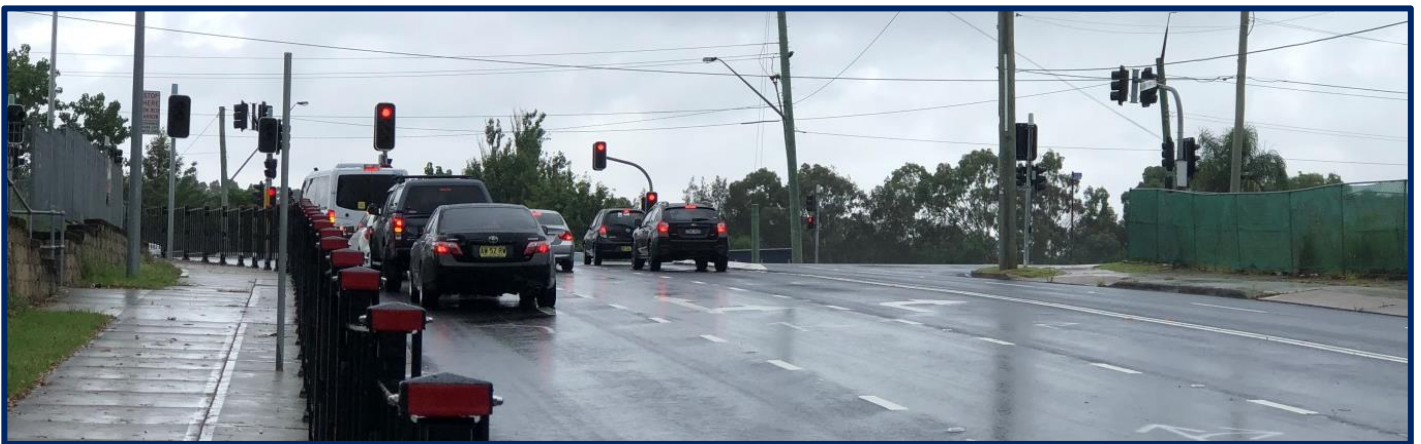
Completed upgrade of Blacktown Road and Great Western Highway intersection
