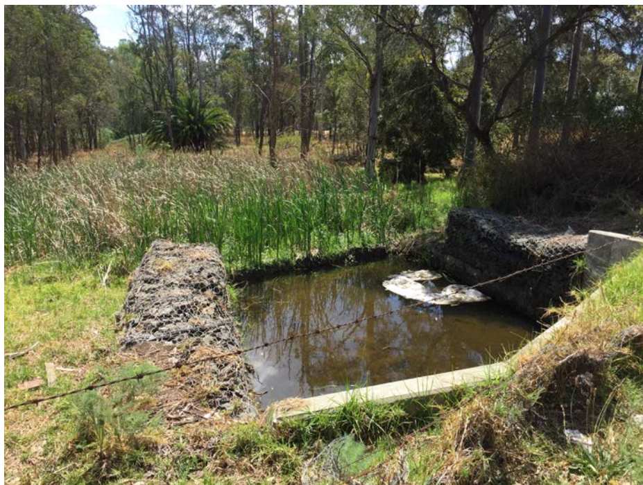
Figure 6-8 Existing culvert outlet (Source: Roads and Maritime Services, 2017)
