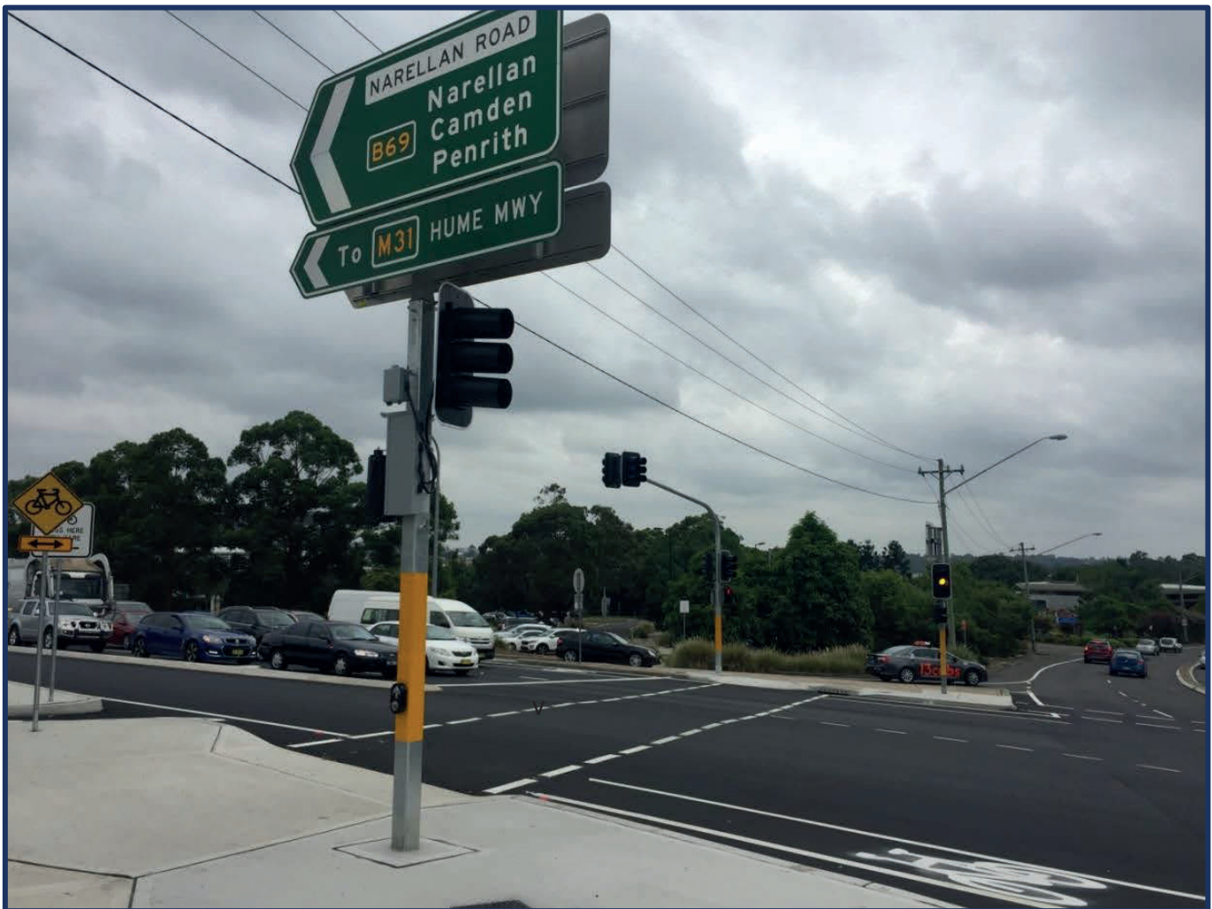
The newly upgraded Narellan Road and Appin Road intersection in Campbelltown
