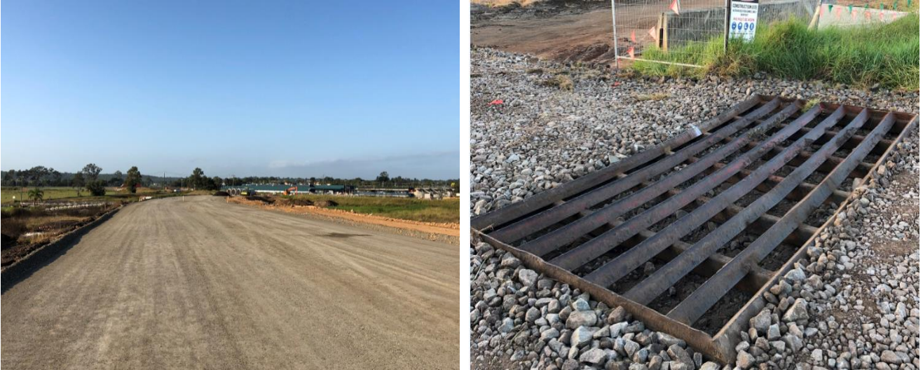
Figure 10 SMZ placed at fill 1 (left) stabilised access and egress points (right)
