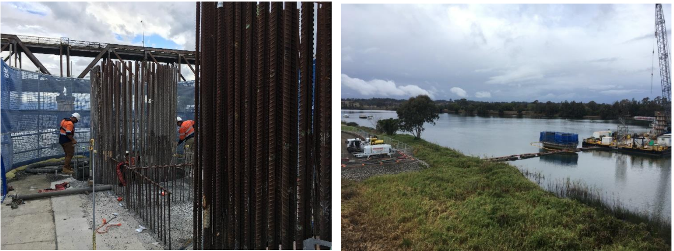
Figure 7 hydro demolition at pier 6 with effective controls in place
