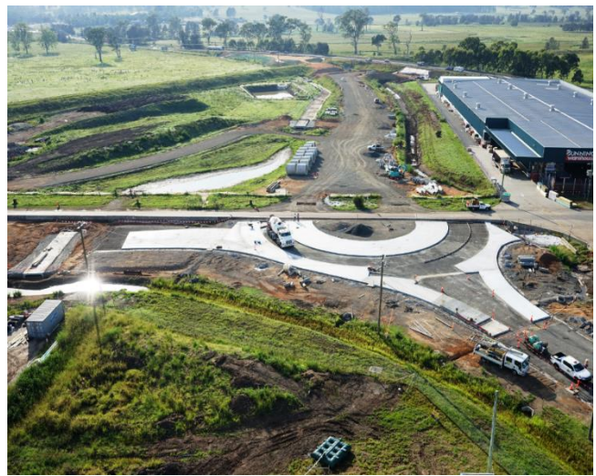
Figure 1 Seal and subsoils place on fill 2 (left) and construction of the new roundabout at Iolanthe and Through Street (right)
