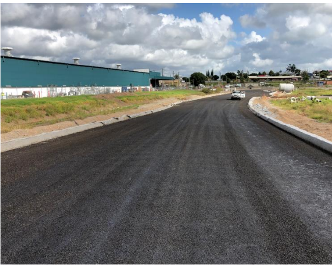
Figure 1 Seal and subsoils place on fill 2 (left) and construction of the new roundabout at Iolanthe and Through Street (right)
