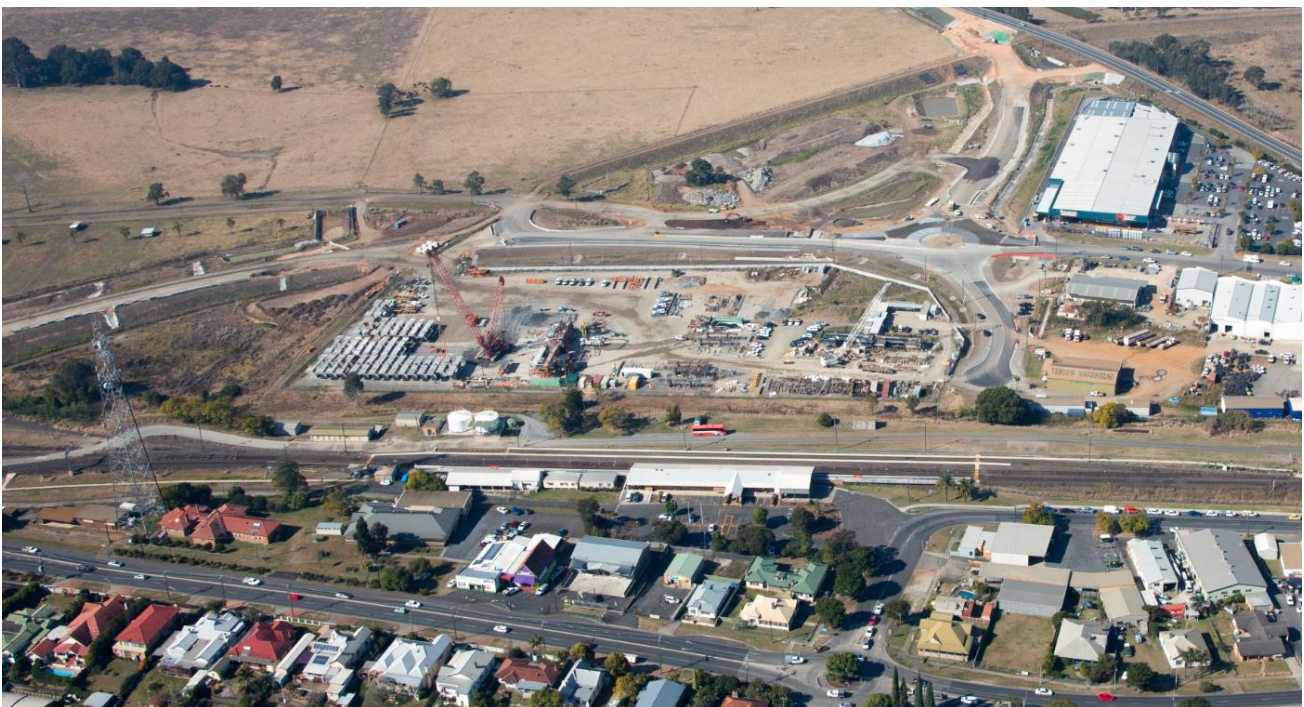
Figure 5 Aerial photo of the South Grafton casting yard
