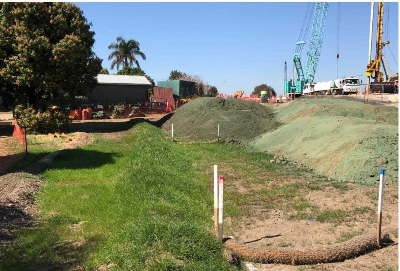
Figure 11 Grass strike and controls installed near abutment B in Grafton
