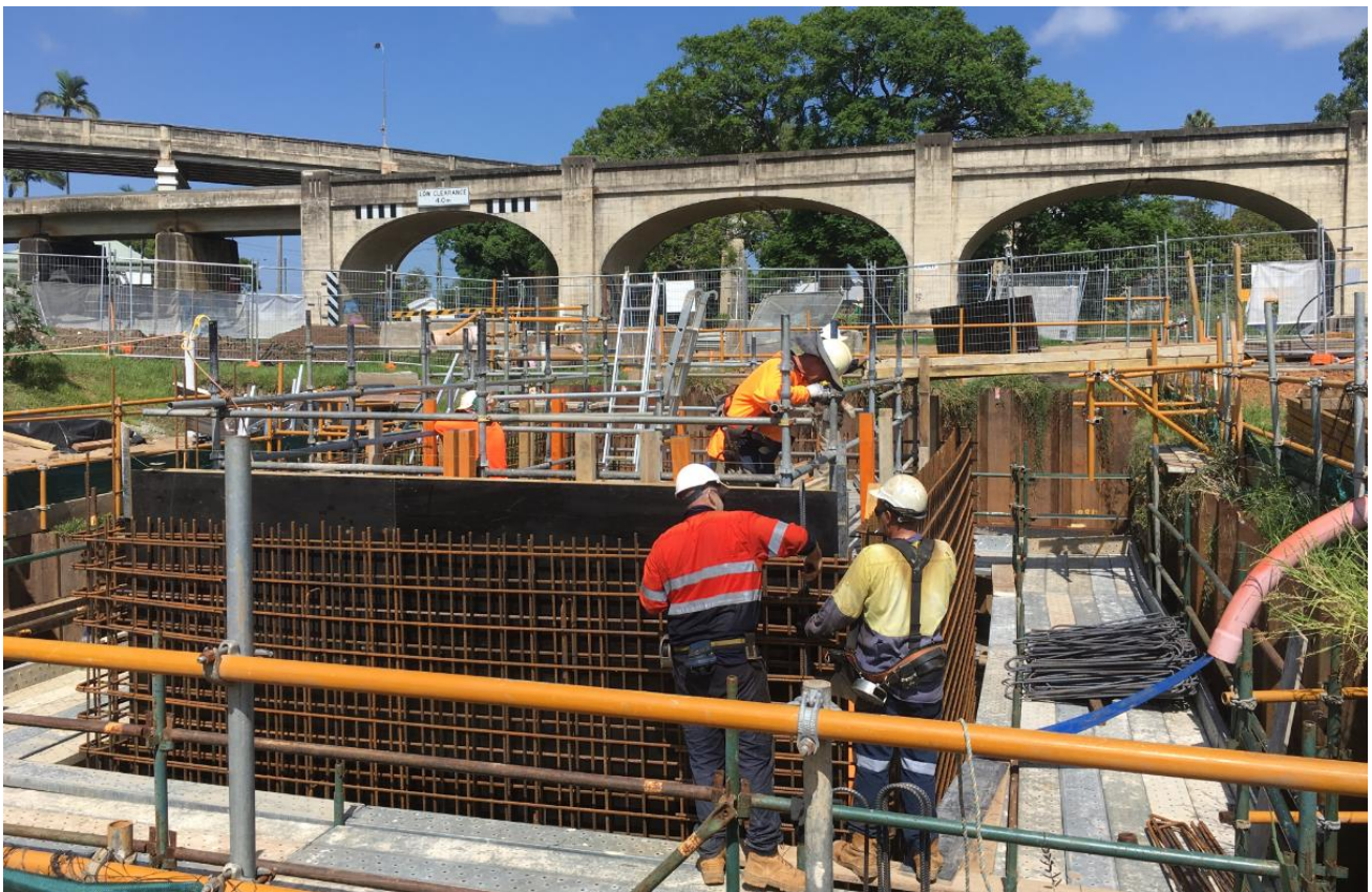
Figure 1 Form work and steel tying setup at the Grafton pump station
