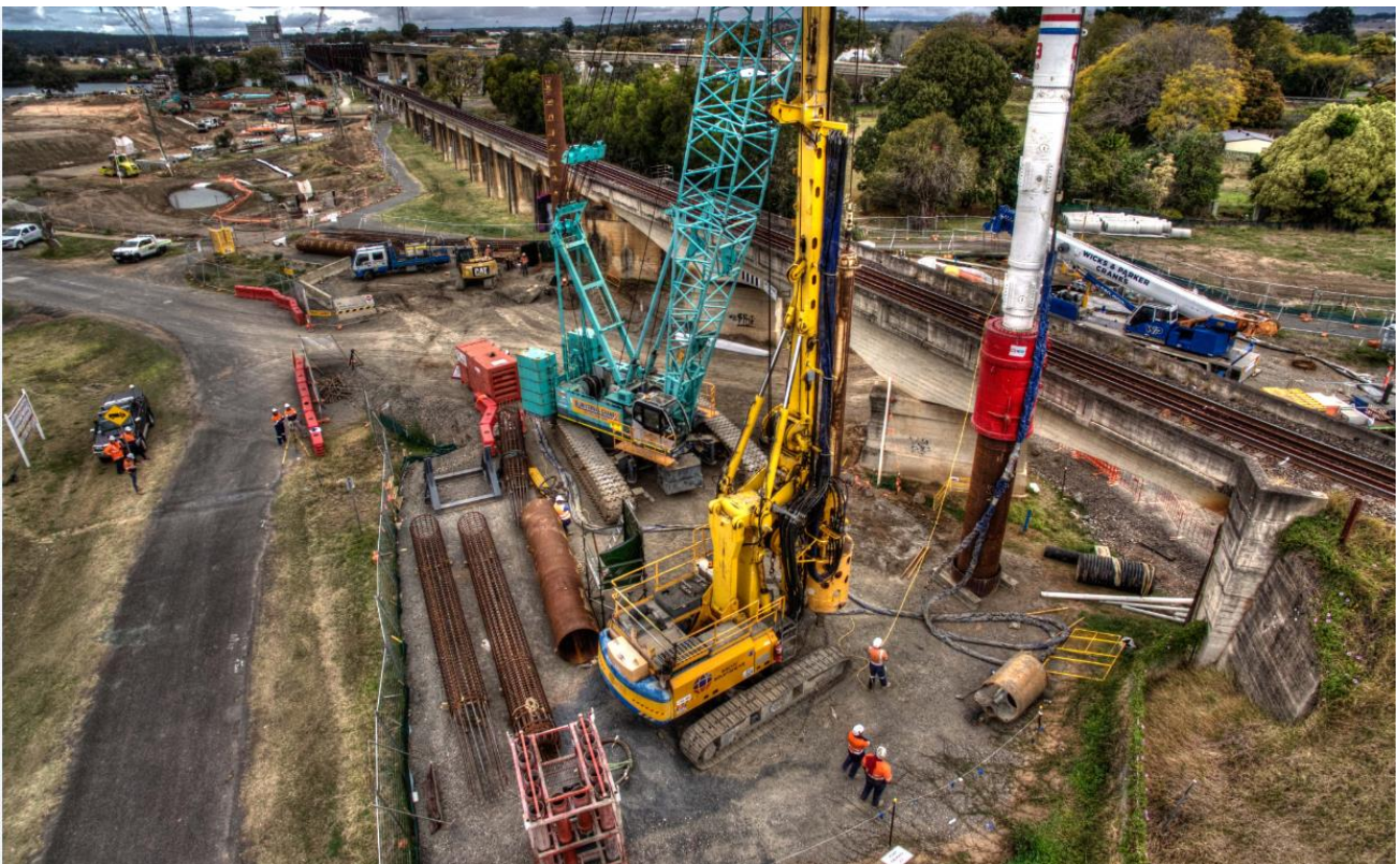
Figure 8 Piling works at the Rail bridge completed in the reporting period
