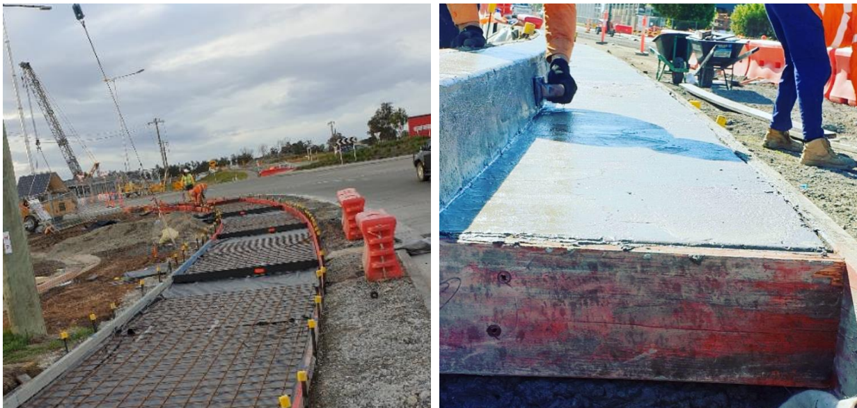
Figure 9 Completion of footpaths and kerb
