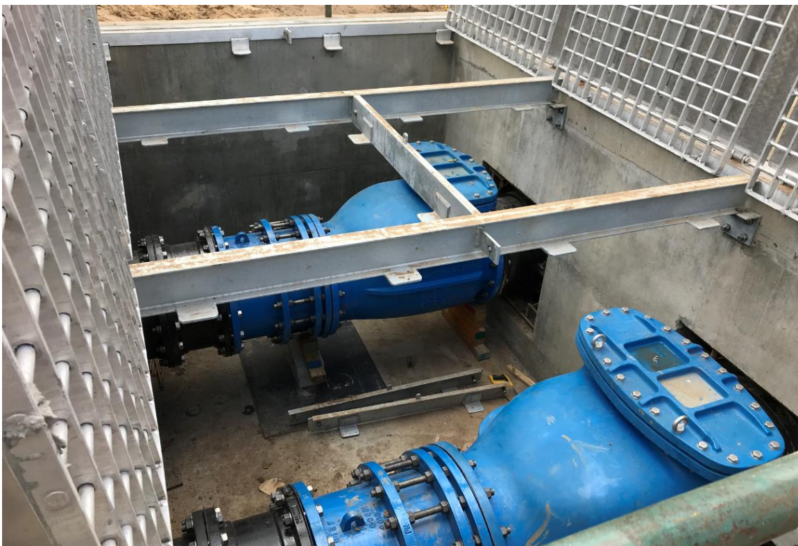
Figure 1 New pump infrastructure installed into the Grafton pump station
