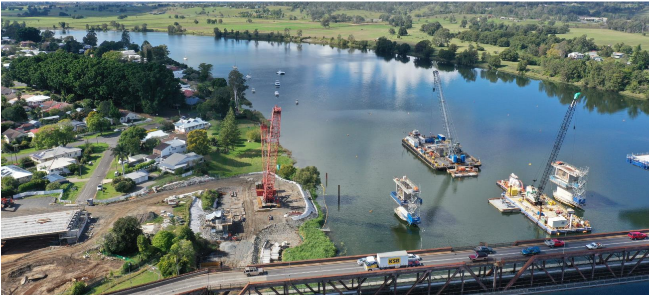
Figure 7 Marine works progress
