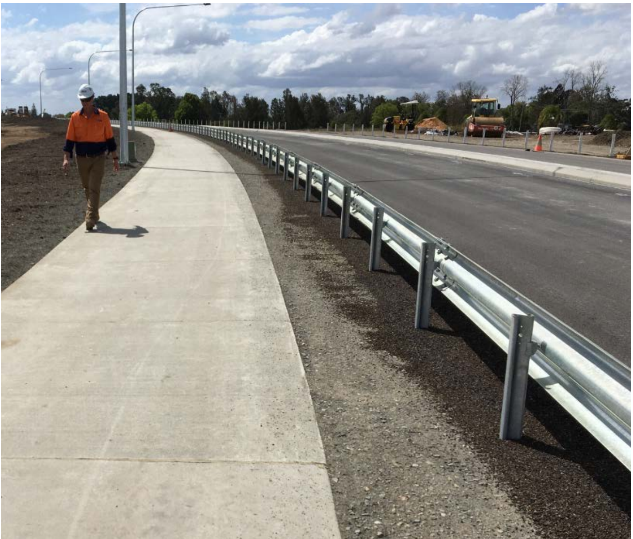
Figure 3 fill 1 finalised verge, steel barrier, street lighting and asphalt
