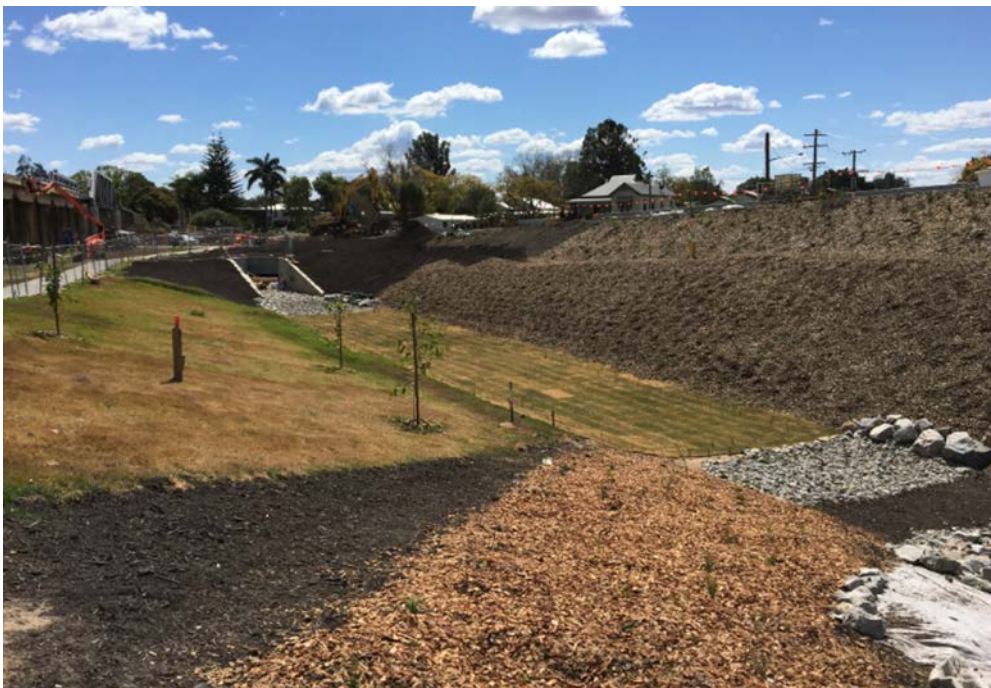
Figure 9 Completion of landscaping and final drainage features
