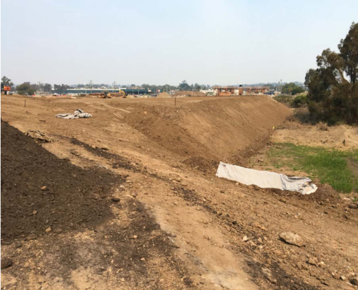
Figure 8 beneficial reuse of surplus material in south Grafton to improve land use
