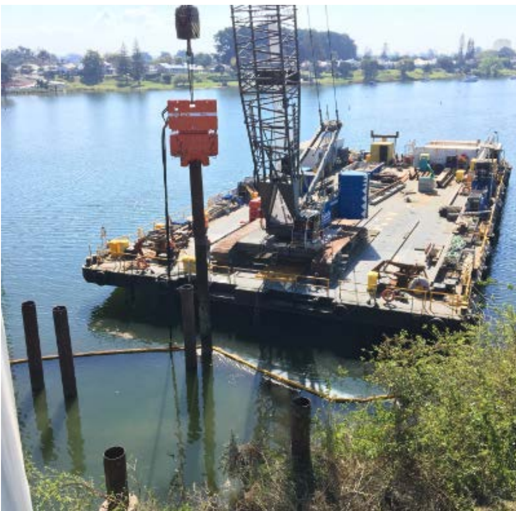
Figure 5 Removal of the temporary jetty in south Grafton
