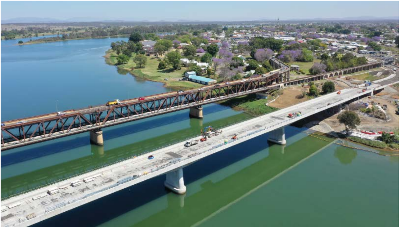
Figure 7 Marine works progress
