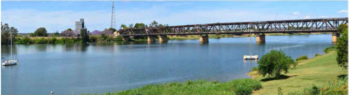
Figure 15: Existing view looking upstream
