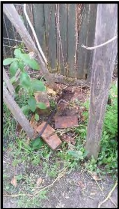
Plate 8-4. Capture location at APO 13 with brick displaced.
