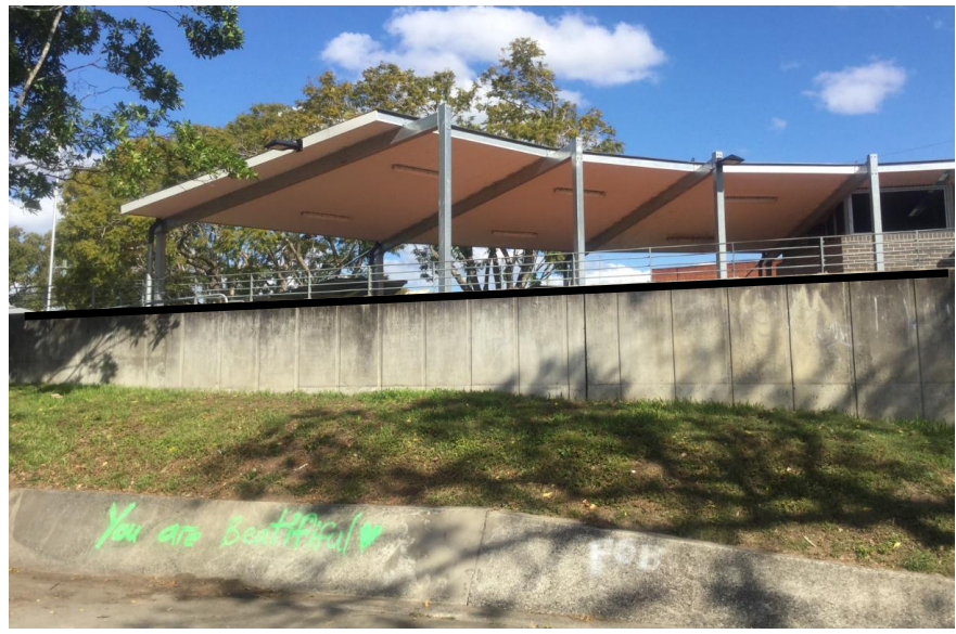
Example scenario 5: Concrete block wall height extension shown by the black line. Remove all waste materials, control cementitious material, do not store chemicals at the site remove each day.
