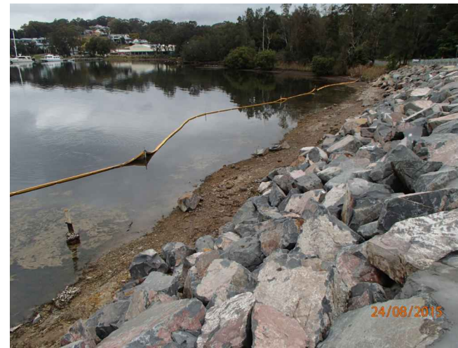
PHOTO EXAMPLE 7 - SILT CURTAIN
