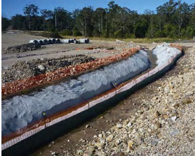
Figure 3. A geofabric lined temporary clean water diversion traversing a work zone during installation of cross drainage. The geofabric has been anchored at the top with star pickets at regular intervals. The star pickets are also integral to sediment fencing preventing sediment from entering the channel along the length of the diversion. Within the channel larger rock is used to aid in energy dissipation. Orange safety fencing effectively delineates the diversion and allows.
