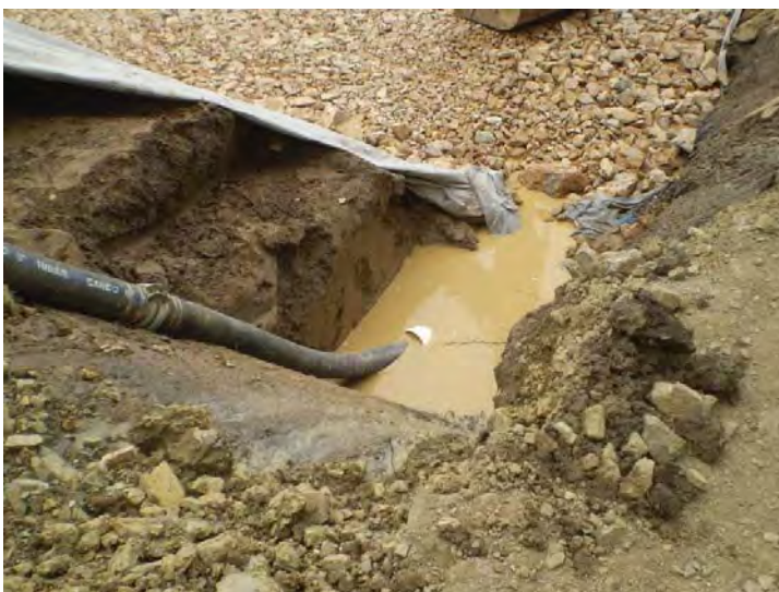
Figure 4. A sump adjacent to a working area may require higher levels of maintenance in order to remain effective. Dewatering to a larger sediment basin will be a more viable treatment measure when compared to flocculating the sump itself. Consideration to minimising exposed fines around the immediate catchment (e.g. bottom left corner of the figure) will also reduce sediment entering the sump if deemed practical for construction purposes.
