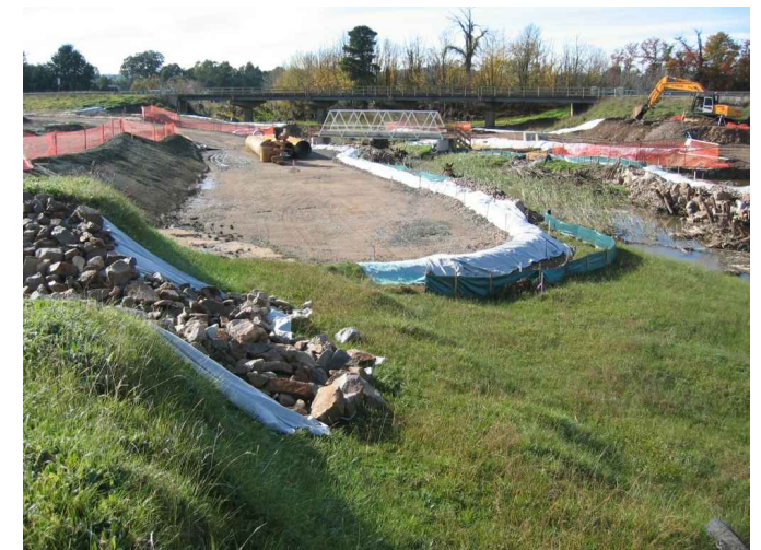
PHOTO EXAMPLE 8 - ROCK PILING PLATFORM
