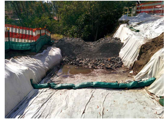
PHOTO EXAMPLE 6 - EXAMPLE OF ROCK FILTER DAM AND SUMP
