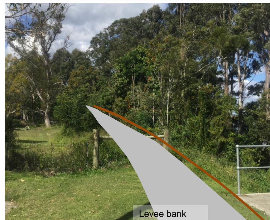
Example scenario 2: Earth embankment area controlled with a mulch windrow produced during clearing
