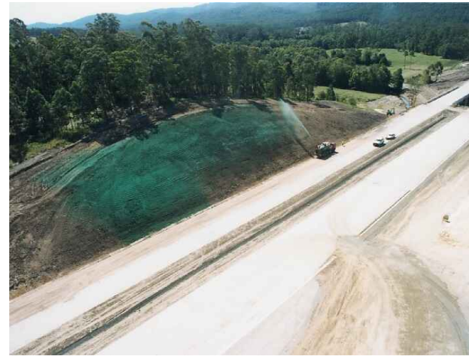
PHOTO EXAMPLE 5 - STABILISATION OF BATTERS
