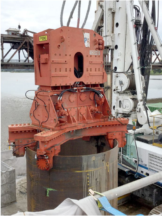
Piling hammer vibrating a steel casing into place
