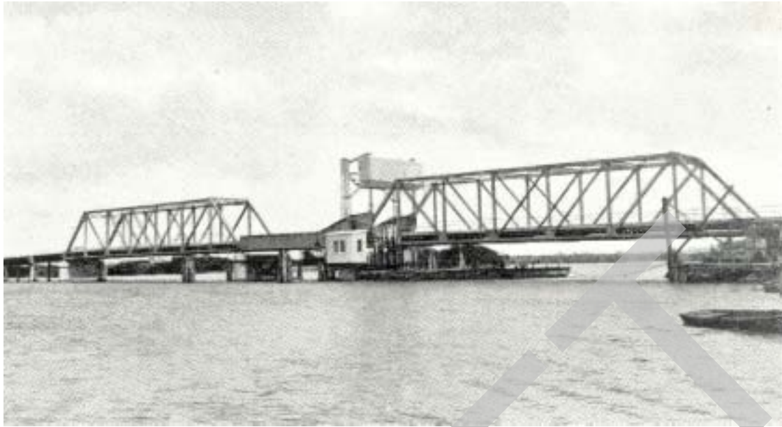
Figure 4: View of Barney's Pont Bridge looking west (DMR, 1953:89).
