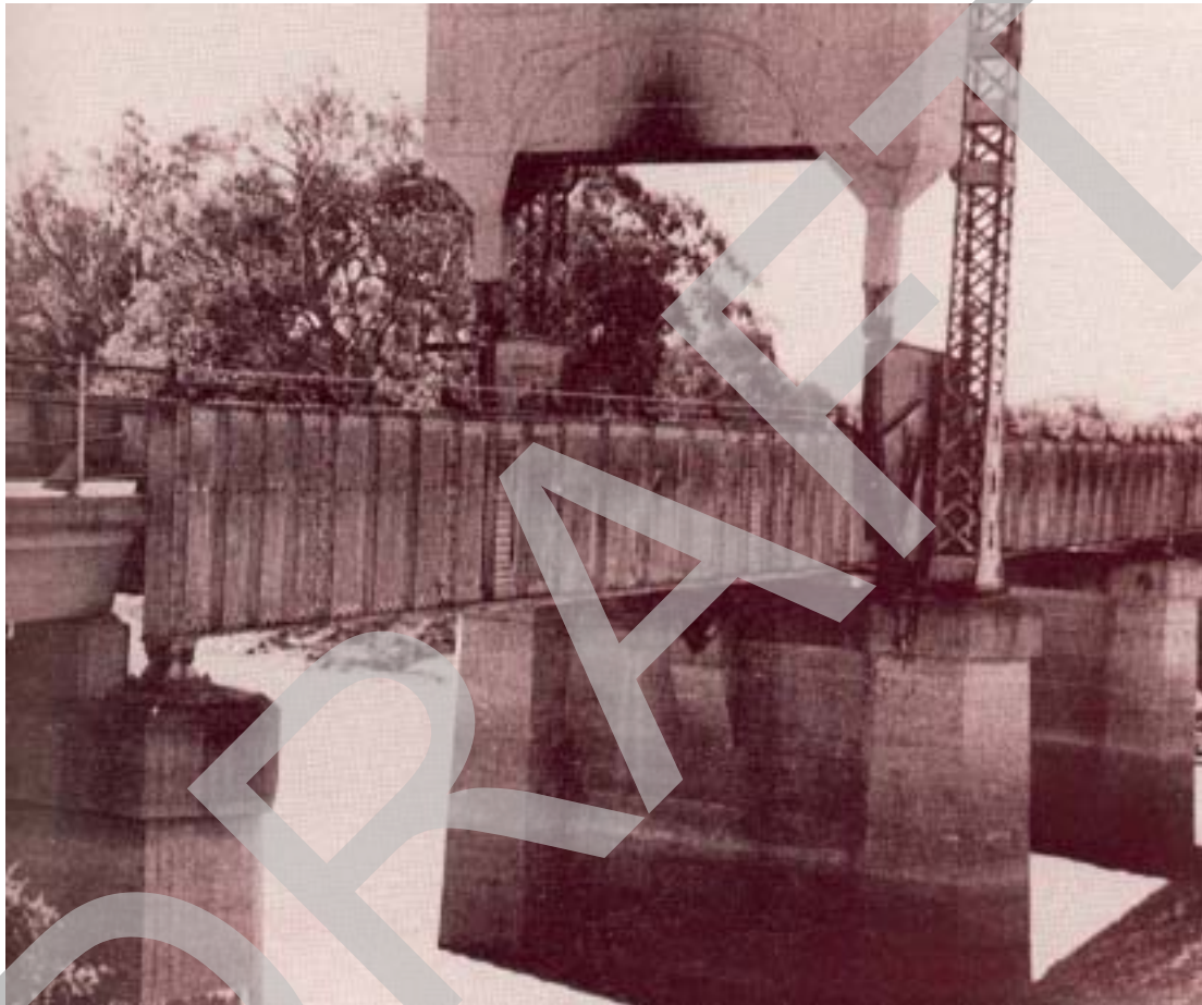
Figure 3: View of the Menindee Bridge in 1958 showing the concrete counterweight and the associated towers that have since been removed (DMR, 1977:7).
