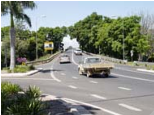
Illustration 24 – the northern approach to the Clarence River Bridge
