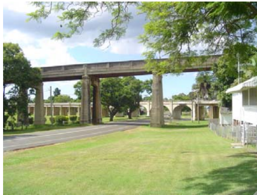
Illustration 4 – northern approach to the bridge
