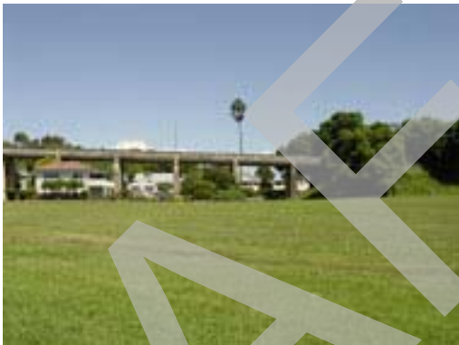
Illustration 25 – side view of the planted embankment
