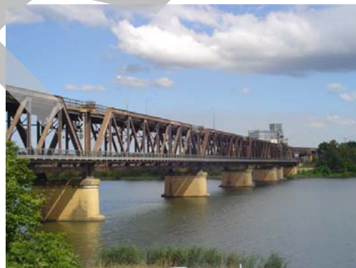
Illustration 3 – view of the Clarence River Bridge from the river end of Fitzroy Street
