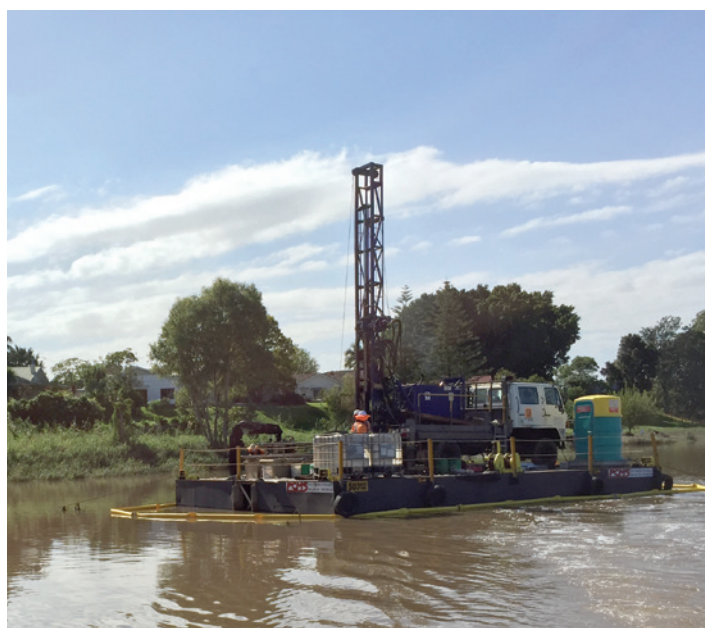
Geo-tech work on the Clarence River
