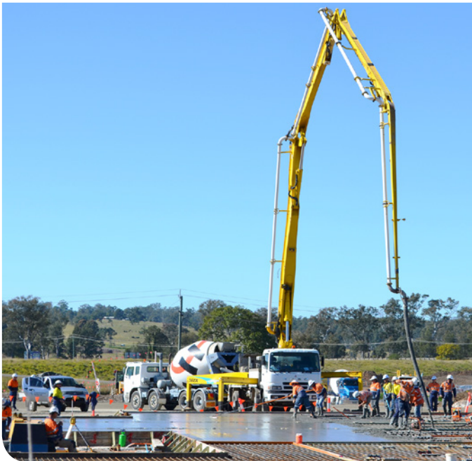
Pouring the concrete slab for the pre-cast facility
