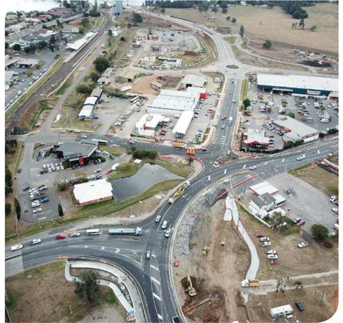
Work has started on the new Gwydir Highway roundabout
