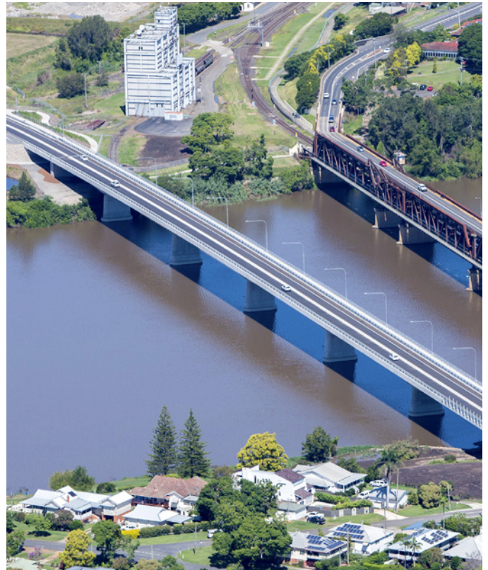
An aerial view of the bridge, looking south
