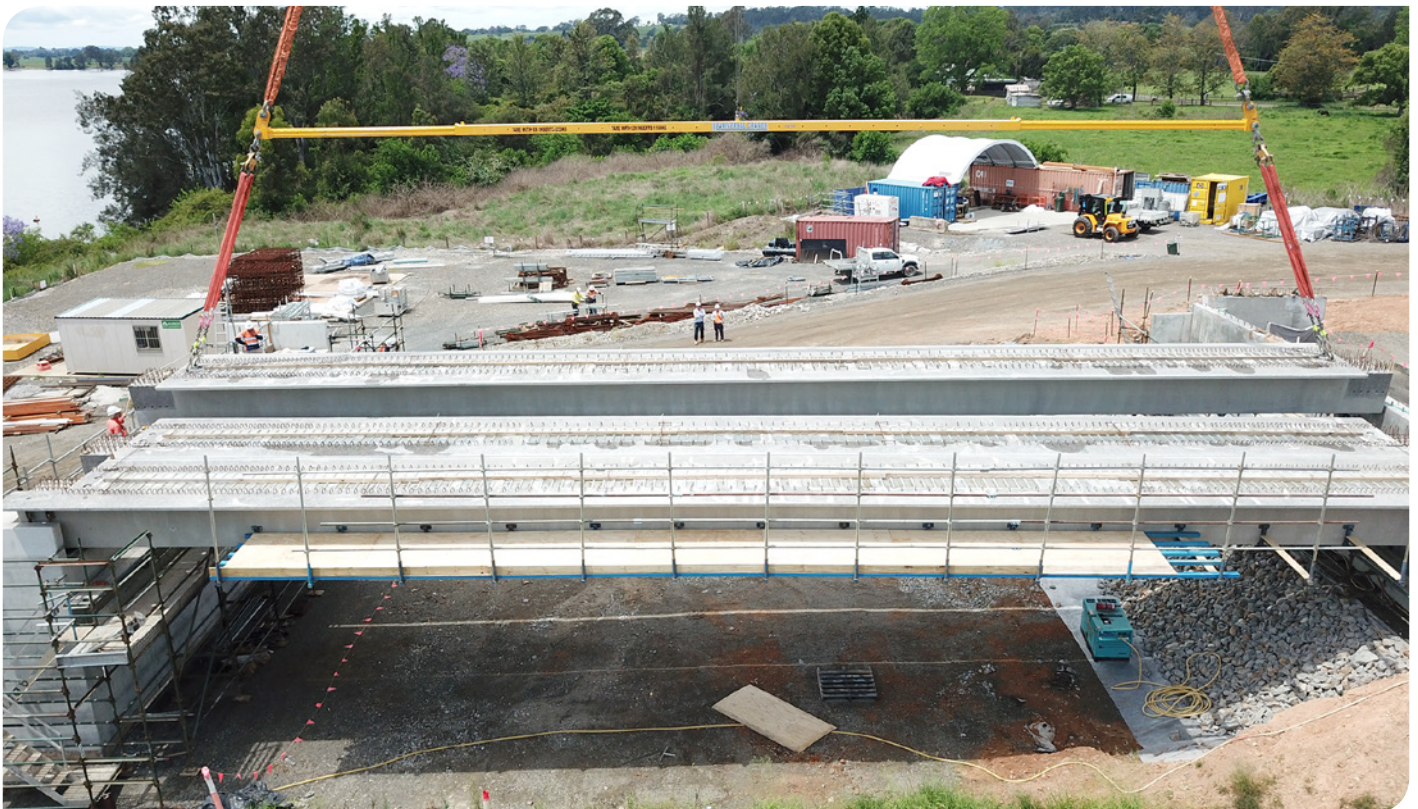
Super-T girders installed at southern abutment, South Grafton (November 2018)
