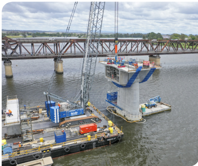
Segment being installed on to pier 3 (December 2018)
