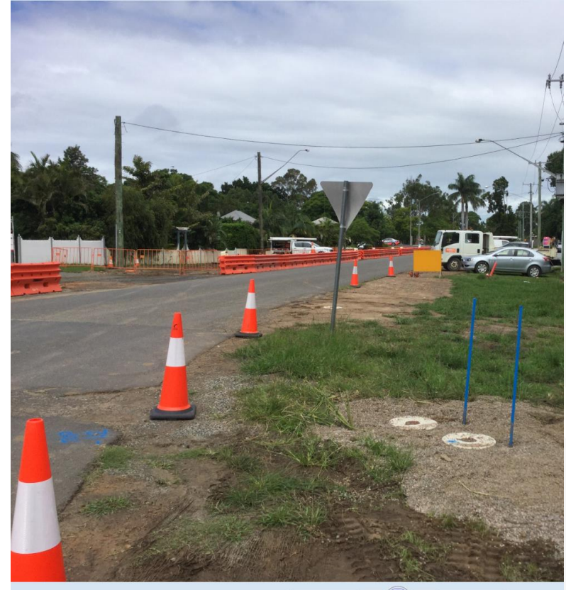
Clarence St Road Construction
