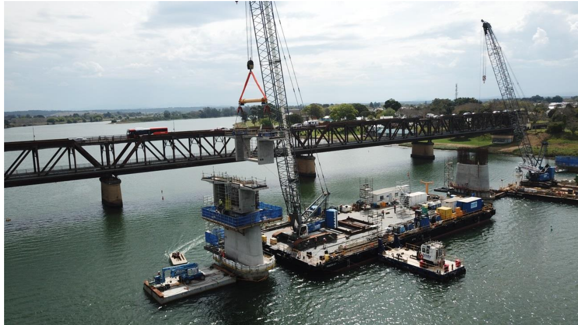
Another segment is lifted into place at pier 4 (October 2018)
