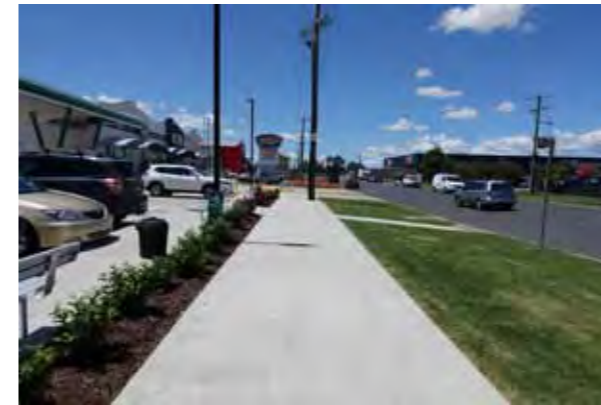
Fig. 5-69: Overhead power line restrict street trees
