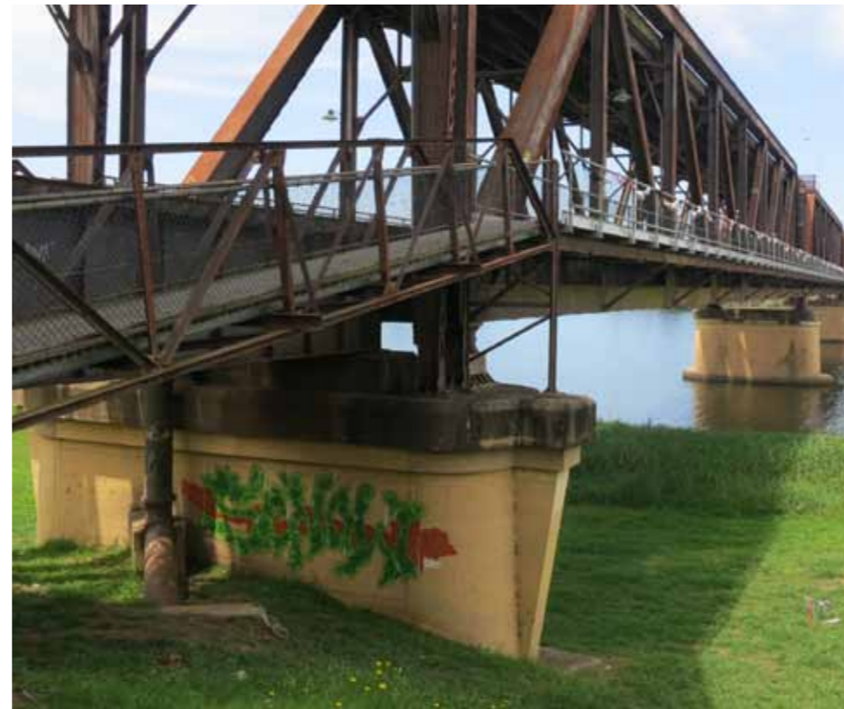
Fig. 5-52: End pier (Grafton side) on existing bridge
