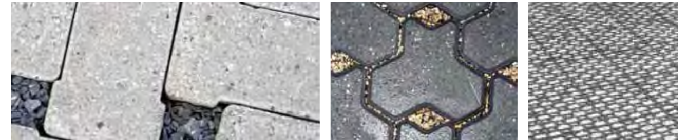
Fig. 5-20: Permeable Paving will be used in areas adjacent existing trees, such as against the Mango trees in Clarence Street
