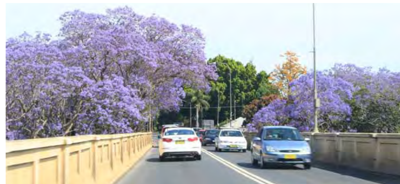
Fig. 1-2: View travelling north on existing bridge
