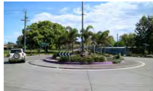
Fig. 2-28: Roundabout on Villiers Street
