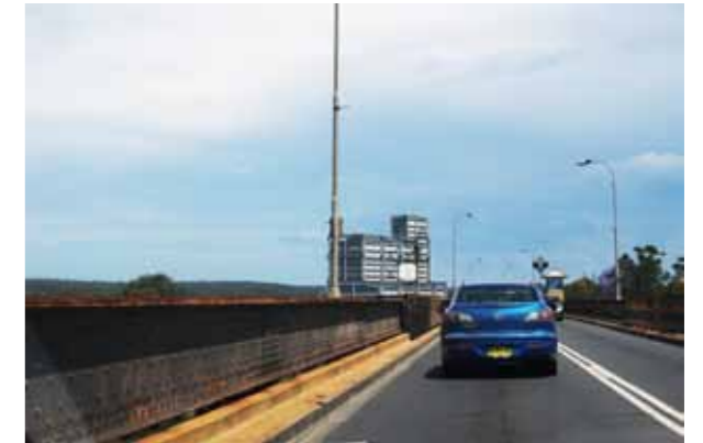
Fig. 2-24: Drivers view from existing bridge looking south
