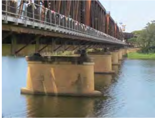
Fig. 4-11: Existing bridge pier form
