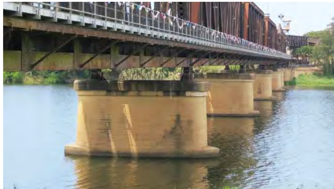
Fig. 2-23: Existing bridge piers
