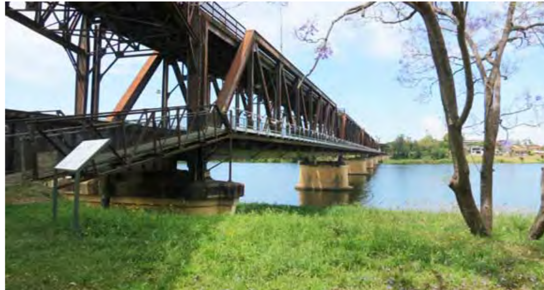
Fig. 2-22: Existing truss bridge over the Clarence River
