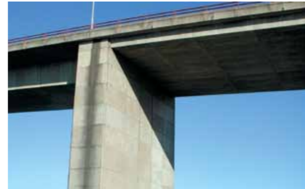
Fig. 4-26: Transition pier example
