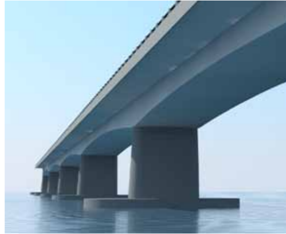
Fig. 4-13: Preferred bridge pier form
