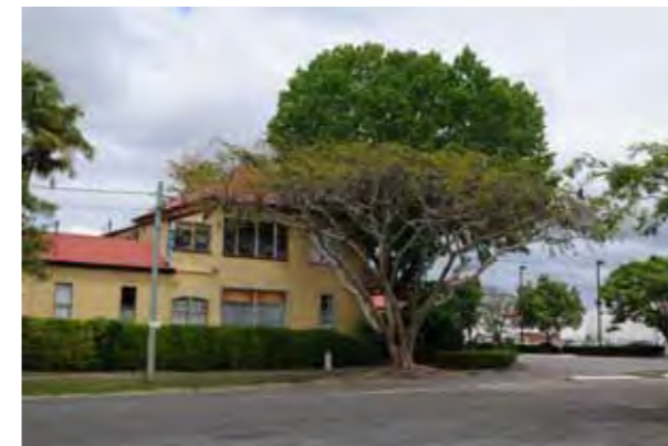
Fig. 5-10: Villiers Street intersection
