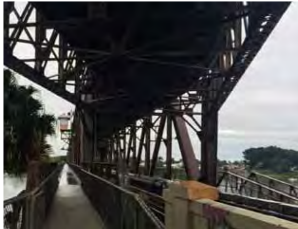
Fig. 4-43: View looking north from South Grafton under the existing bridge.
