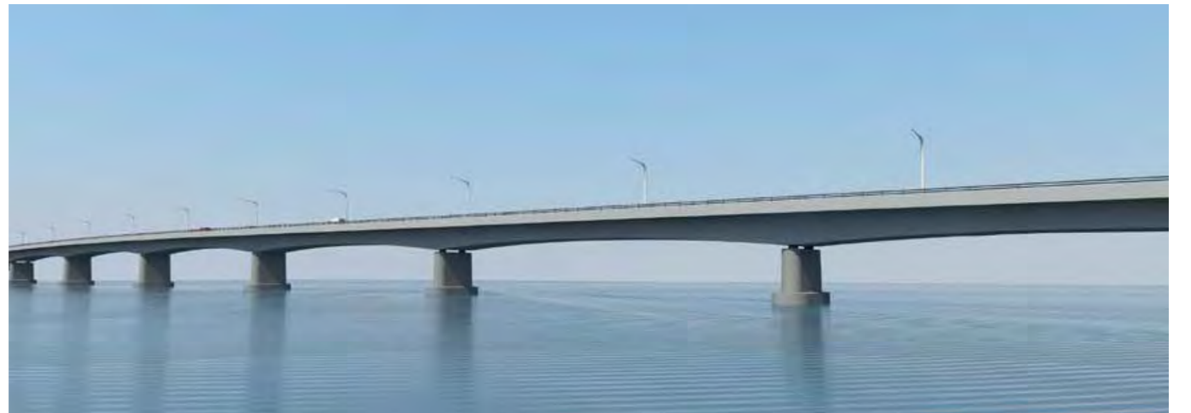
Fig. 4-15: Pier form option - rectangular blade with double chamfers (increasing width)
