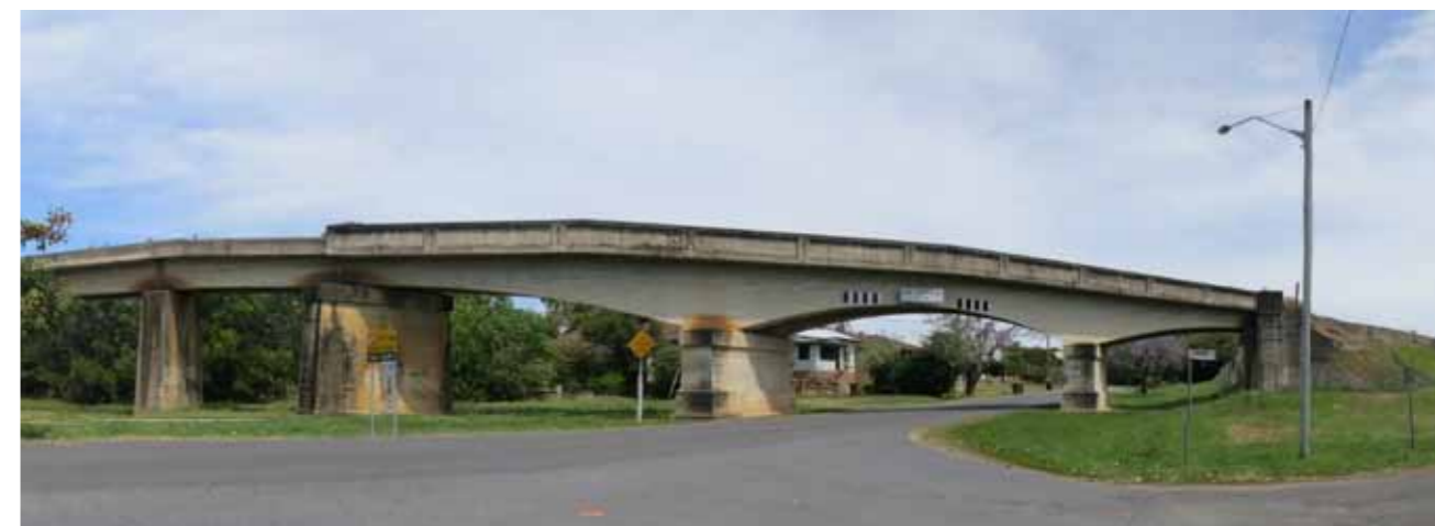
Fig. 4-29: Existing Pound Street bridge form, looking west towards town
