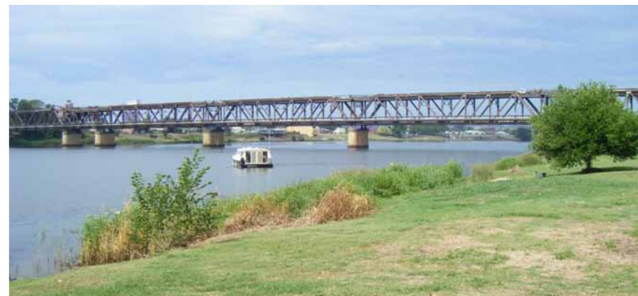
Fig. 1-1: View of the existing bridge looking south west
