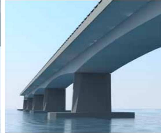
Fig. 4-16: Pier form option - rectangular blade with chamfers
