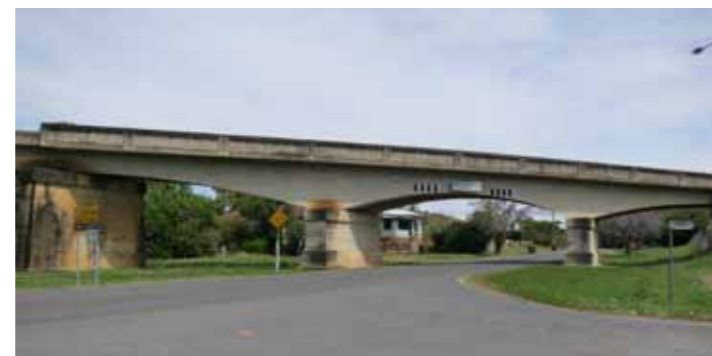
Fig. 5-40: View of existing Pound Street viaduct
