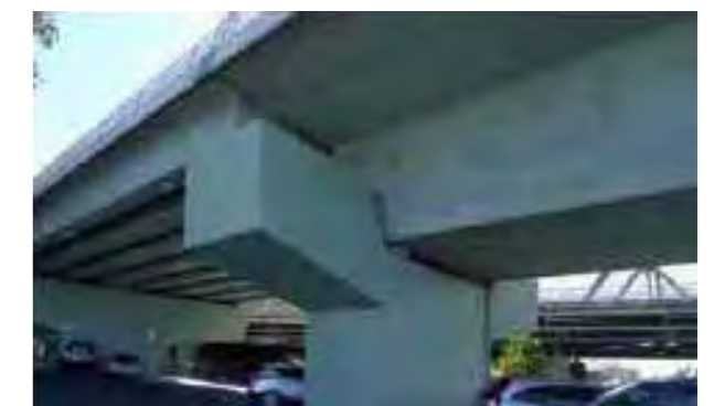
Fig. 4-6: Proposed example of the transition pier - EIS design
