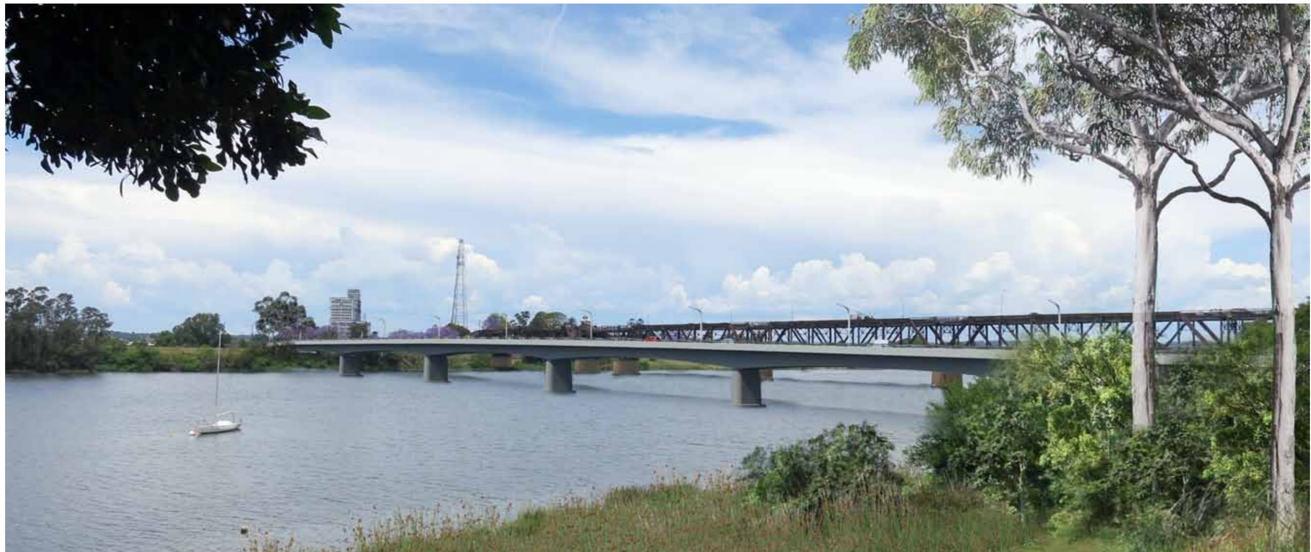
Fig. 5-51: View of the additional bridge over Clarence River at Grafton looking south west
