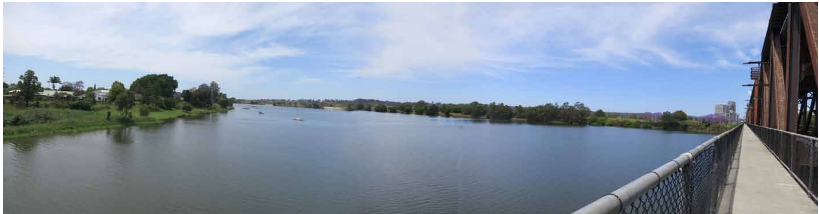
Fig. 5-46: View looking east from the existing bridge
