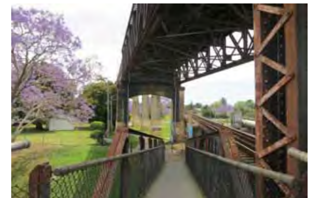
Fig. 2-26: Walkway beneath existing bridge
