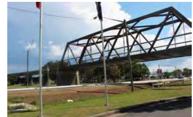
Fig. 2-13: Truss bridge over Gwydir Highway
