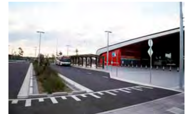
Fig. 4-49: Rain gardens with slotted curb, at Leppington Station, constructed 2015 (design by KI Studio)
