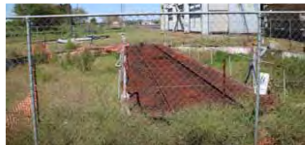
Fig. 8-36: The turntable is a significant heritage element in the context of rail transport in Grafton.
