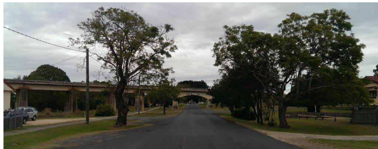
Fig. 8-15: View looking north along Pound Street, to the railway viaduct In the mid-distance. A King George V Plaque on the railway bridge will be relocated, as part of the existing structure will be removed.
