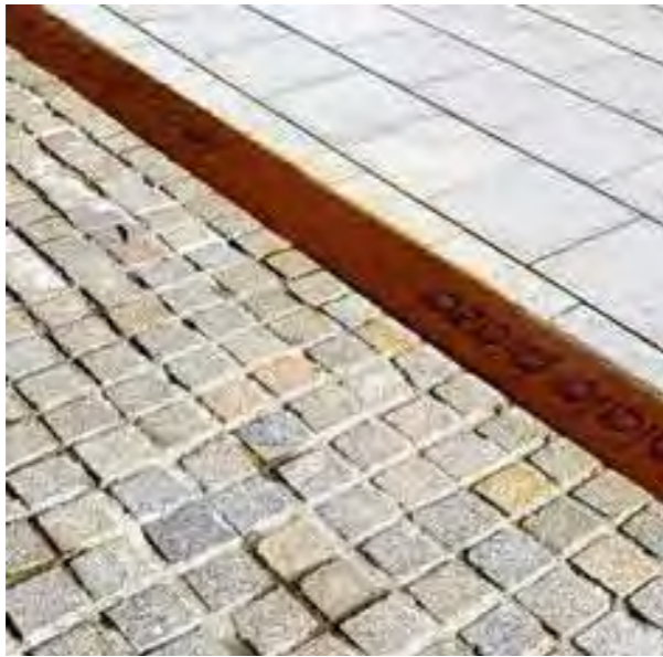
Fig. 8-42: Example of a weathered steel ground inlay without historic references.
