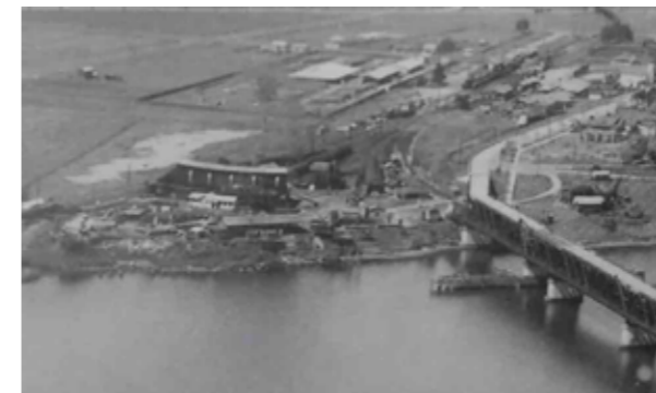
Fig. 8-48: Aerial Image showing the southern riverbank and Locomotive Depot (Source: Comber Consultants, cited in EIS - Appendix G)
