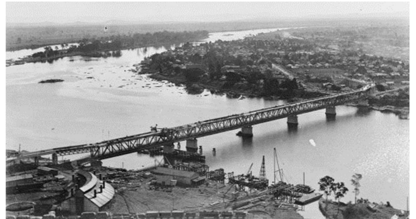
Fig. 8-32: Old photo of the bridge and railway precinct, note turntable to far left. (Source: EIS - Appendix G, p. 51)
