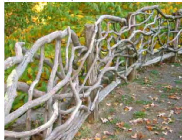
Fig. 8-19: Example of a creative reuse of timber for a railing
