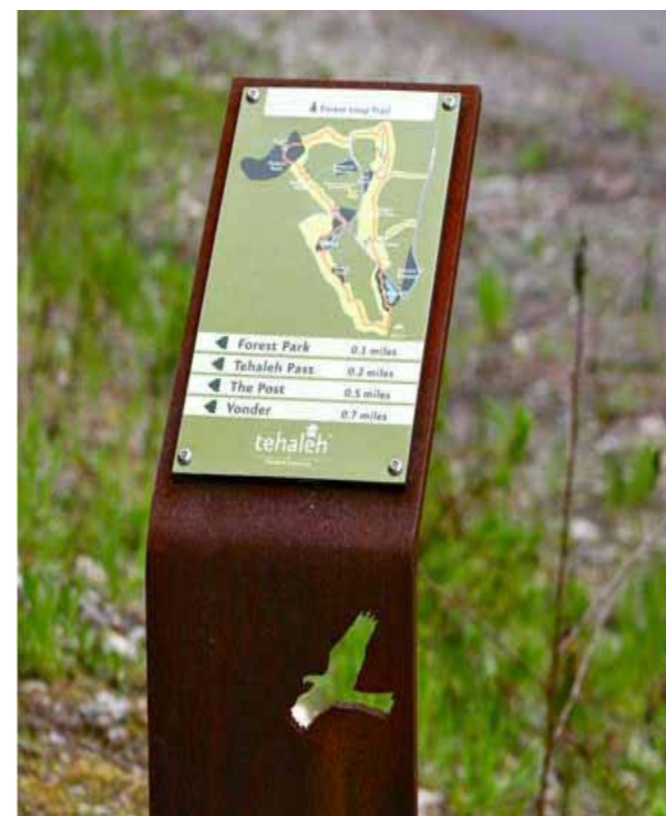
Fig. 8-18: Example of a signage panel using weathered steel. (Source: Drumminhands Design, www.drumminhands.com)
