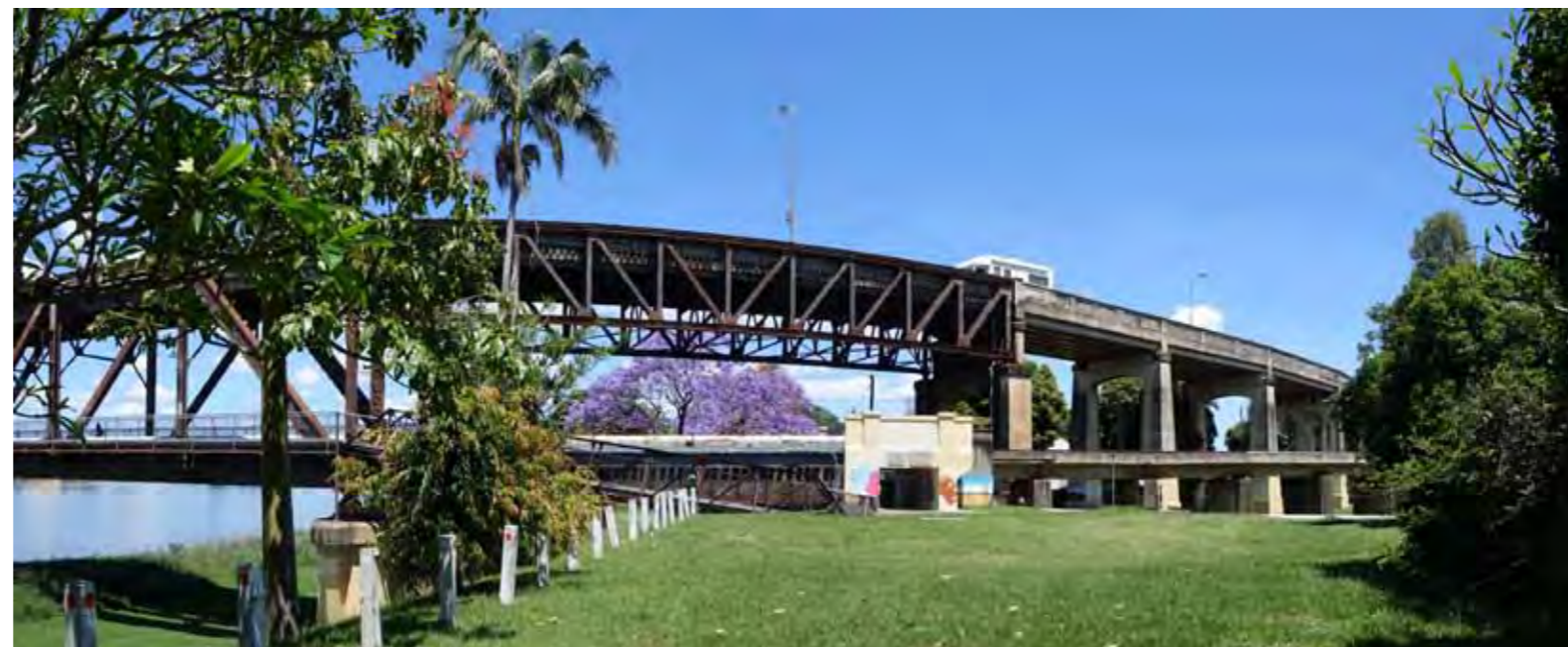
Fig. 8-24: View looking west towards the existing bridge.
