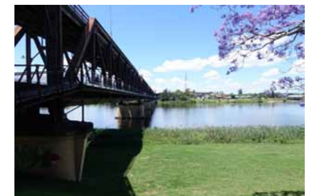
Fig. 8-5: The Old Grafton Bridge crossing the Clarence River
