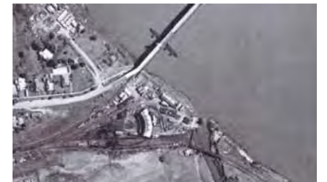
Fig. 8-50: Aerial Image of the South Grafton Locomotive Depot (Source: Comber Consultants, cited in EIS - Appendix G)
