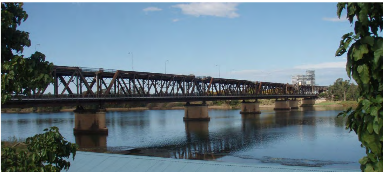
Figure 4: Grafton Bridge from Fitzroy Street
