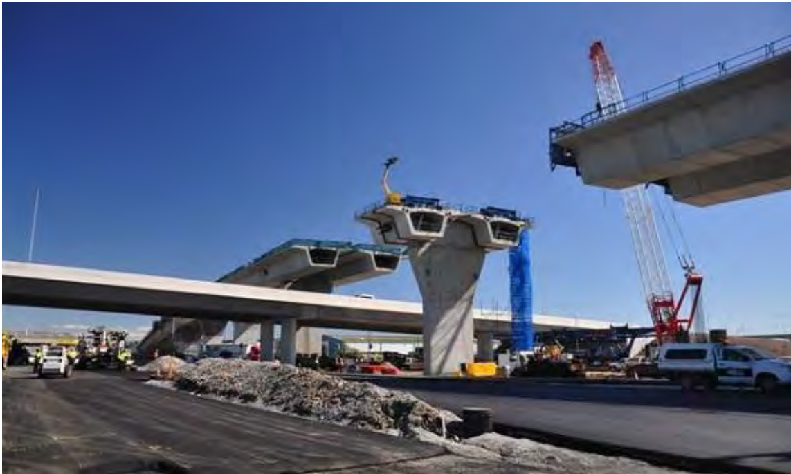
Figure 49: Example of balanced cantilever construction method – Brisbane Airport Roundabout Upgrade (Queensland)
