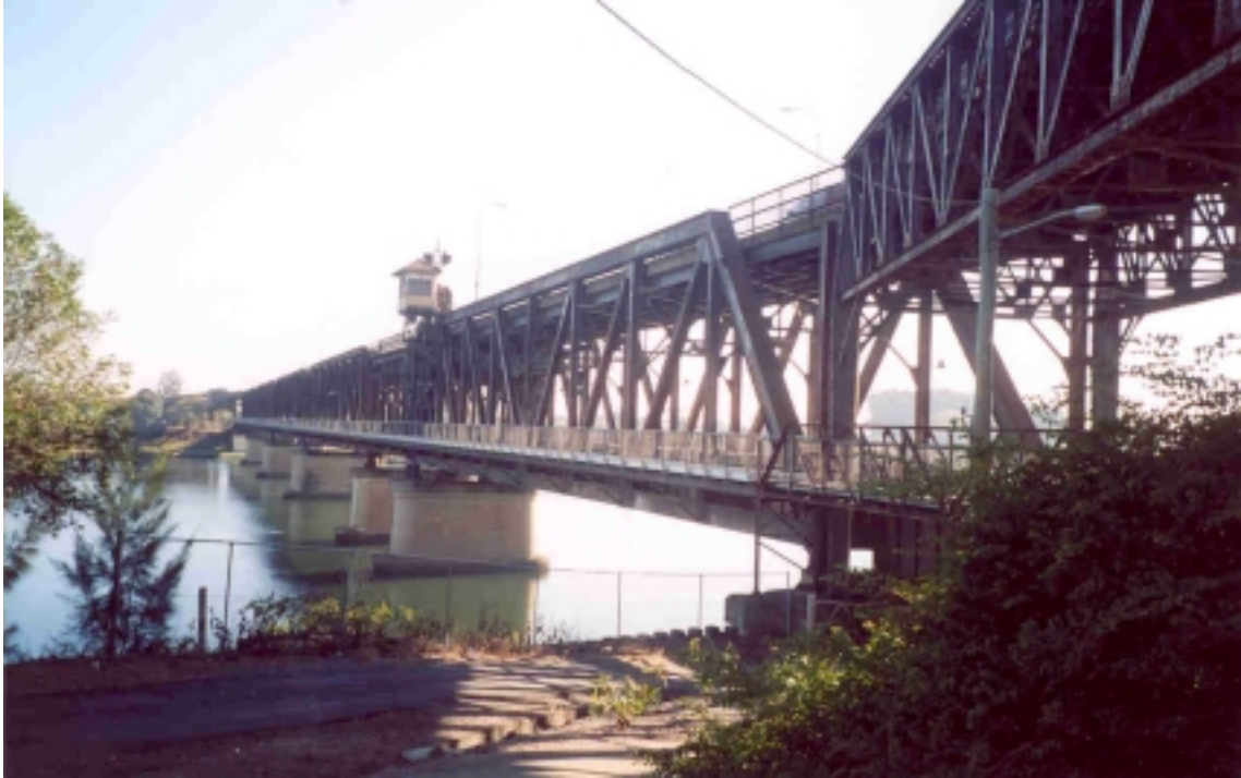
Photo 7 View of existing bridge from South Grafton
