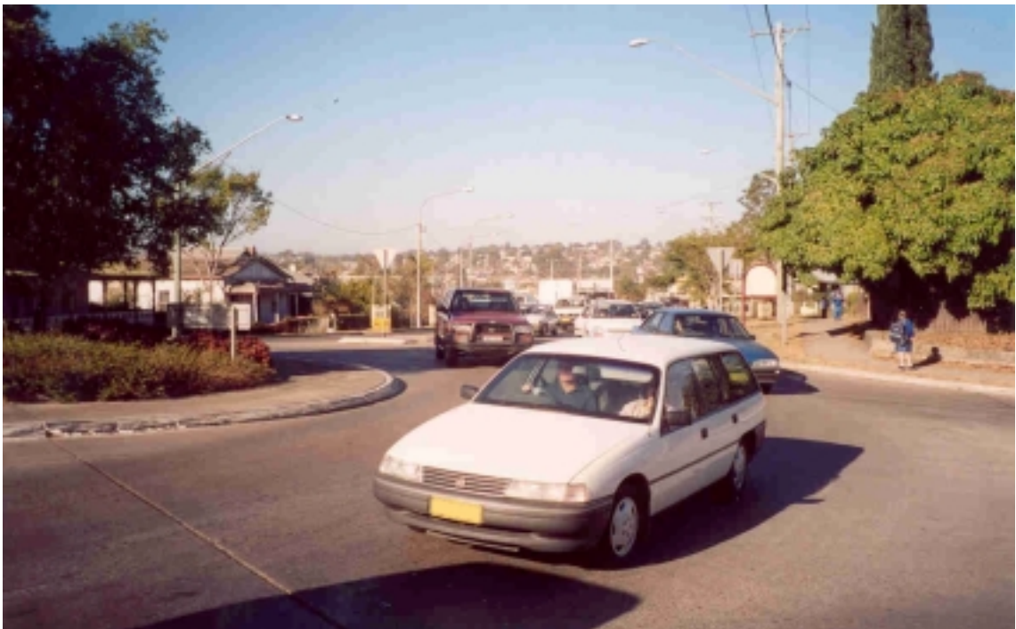
Photo 1 Traffic flow at Through Street roundabout
