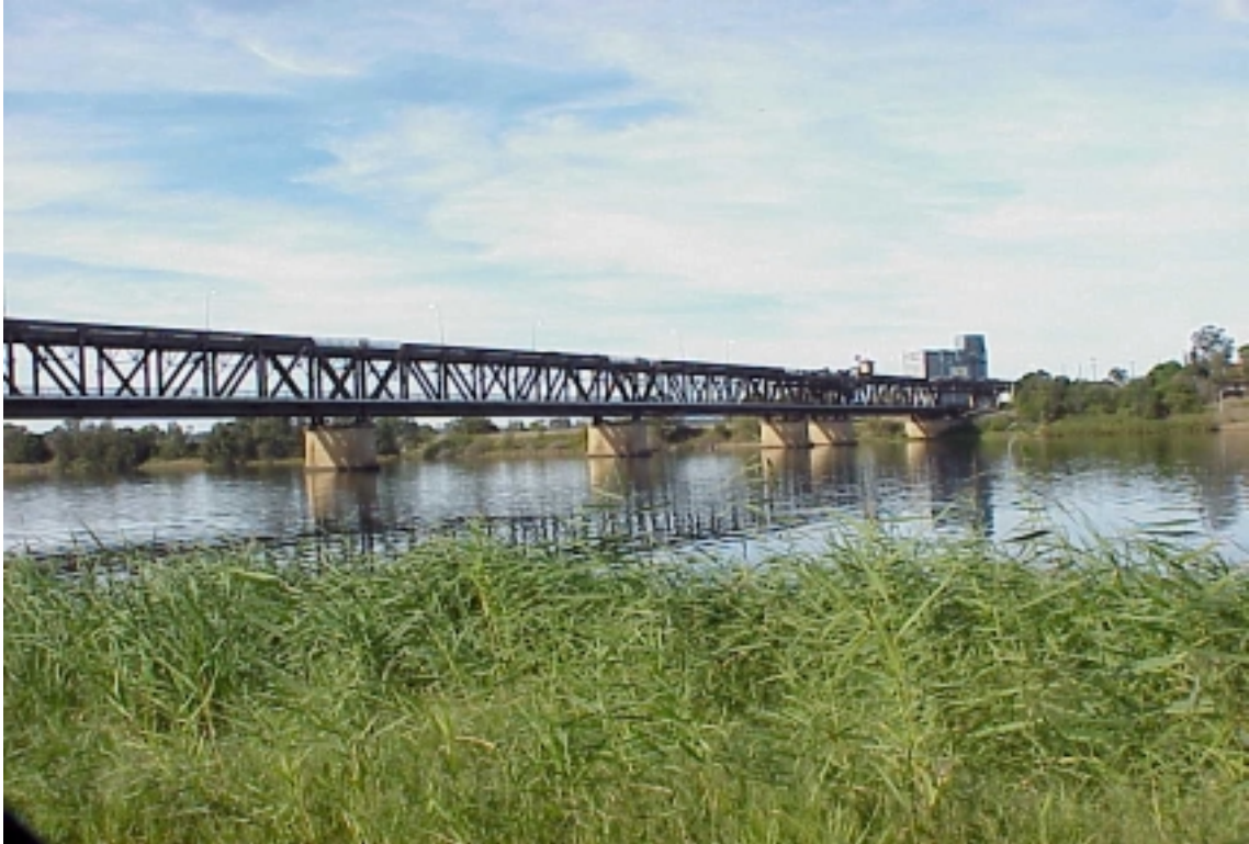
The existing Clarence River Bridge.
