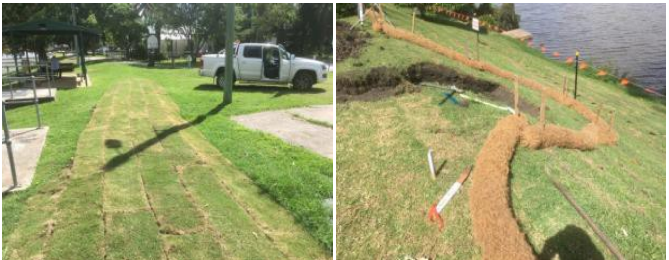
Figure 10 (a), turfing of levee works and 10 (b) coir log controls.
