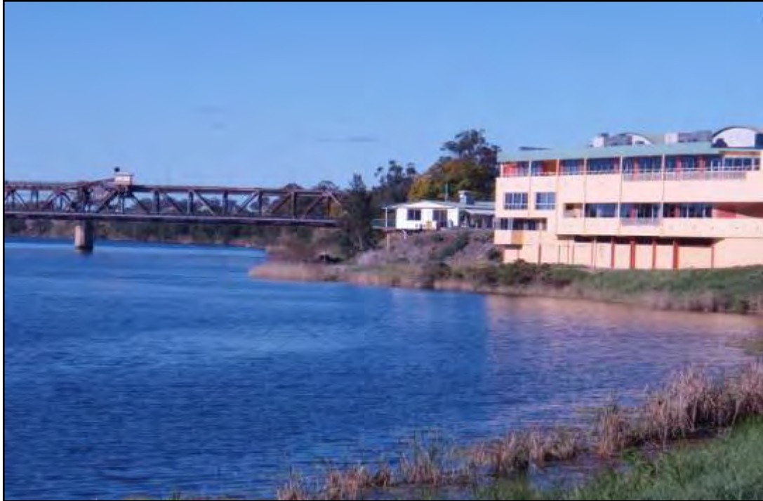
Plate 13: Looking downstream on the southern bank of the Clarence River toward Wharf Street, South Grafton, and the Grafton Bridge.
