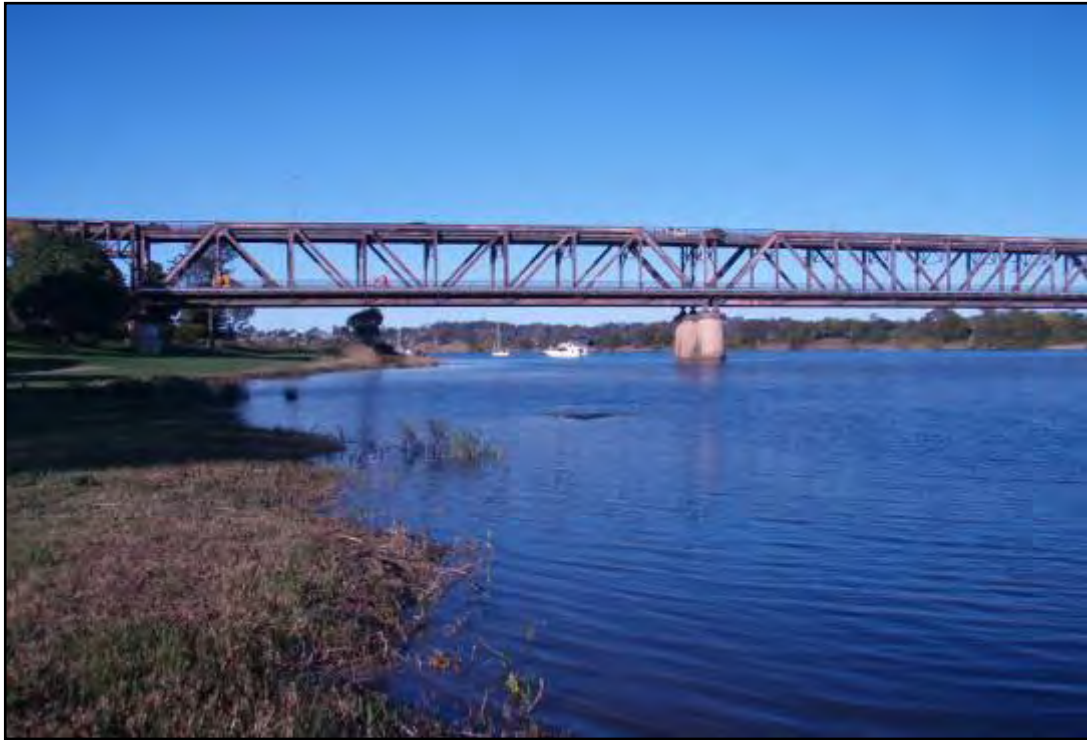
Plate 11: Looking downstream on the northern bank of the Clarence River.
