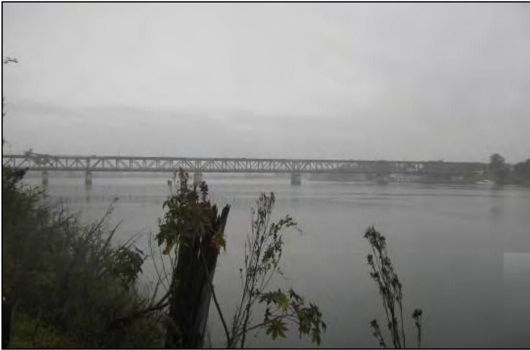
Plate 1: Facing north-west towards Grafton Bridge. Splintered stump in foreground providing potential habitat for microbats.
