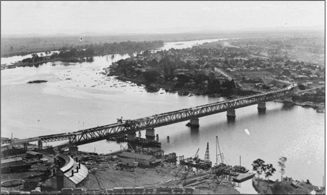
Plate 16: Aerial view of the opening of Grafton Clarence River Bridge, Grafton, NSW, 20 July 1932 (Source: National Library of Australia). This view shows extensive construction facilities on the south bank of the Clarence River and mostly in the project area, the steel siding is visible along with floating pontoons and cranes
