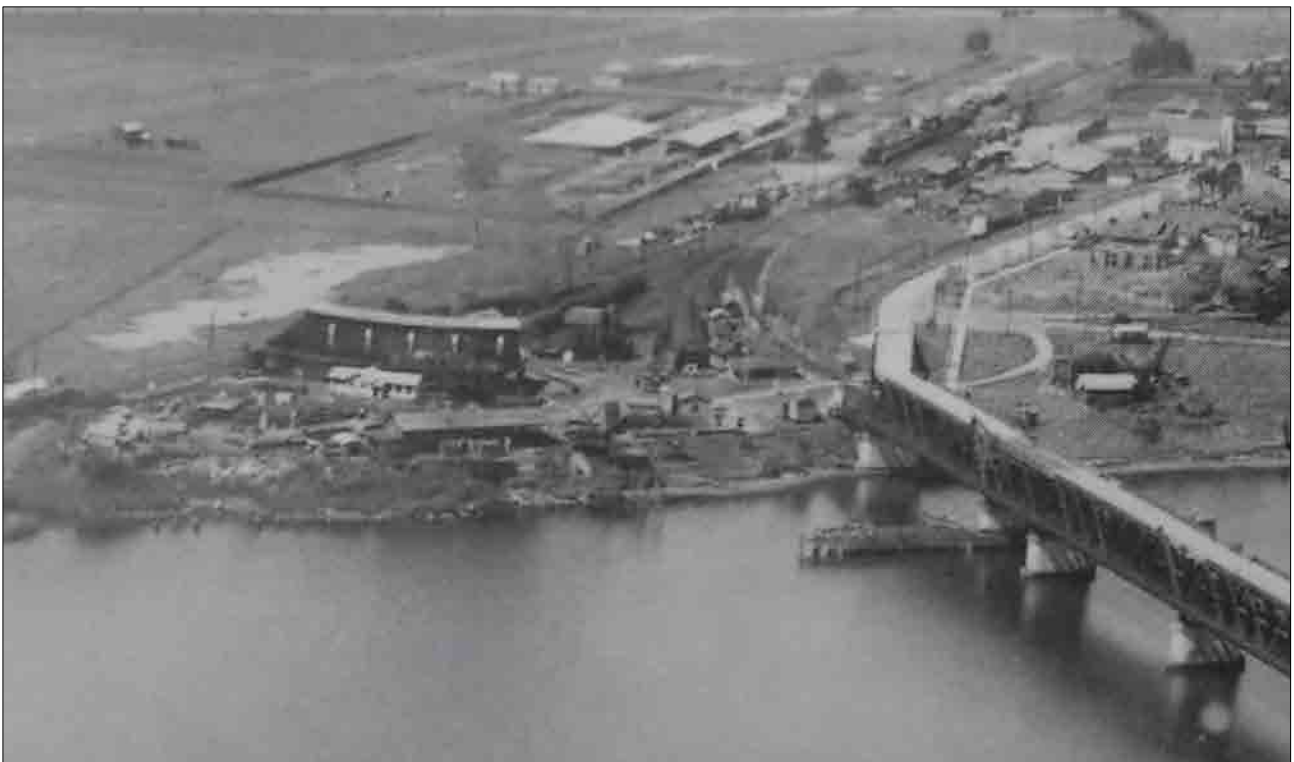
Plate 8: An aerial view of the Clarence River Bridge after construction in the 1930s. Many now-demolished elements of the Railway Terminus area (CZB36 and CZB37) occupy a large area east of the bridge.
