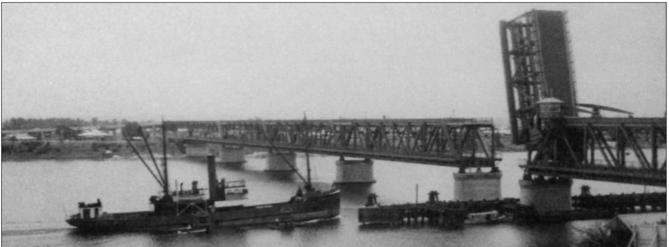
Plate 15: Shipping passing through the bascule span of the completed Grafton Bridge (Source: Kass 2009 p.226)
