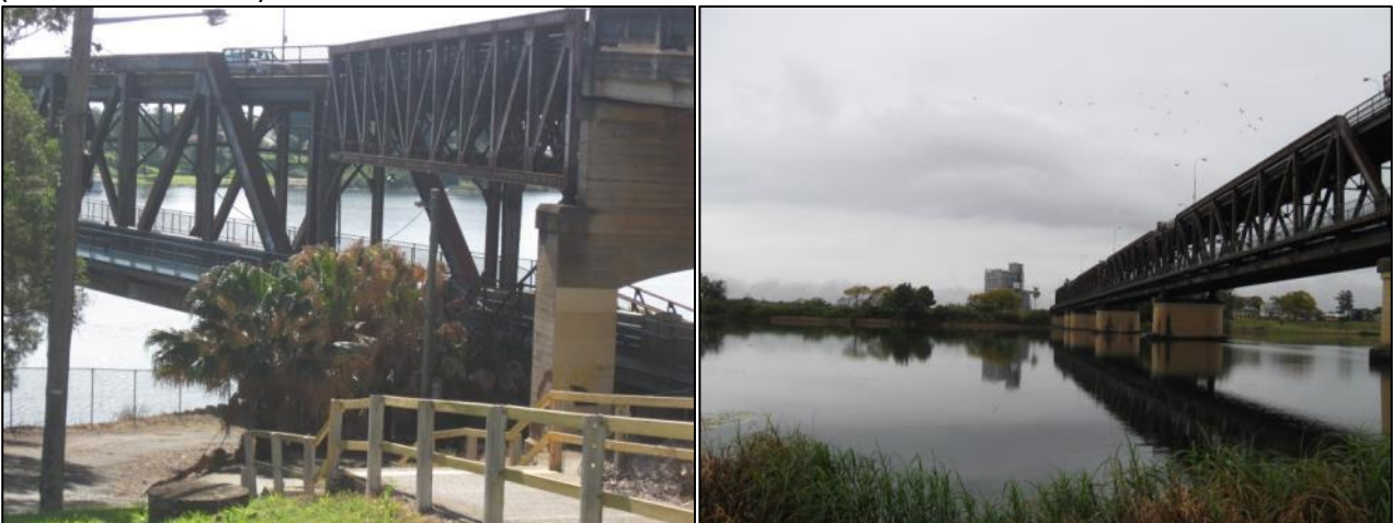
Plate 34: CZB36, north-east facing photograph of Grafton bridge (right) and south-west photograph (left). (Source: Biosis 2012)
