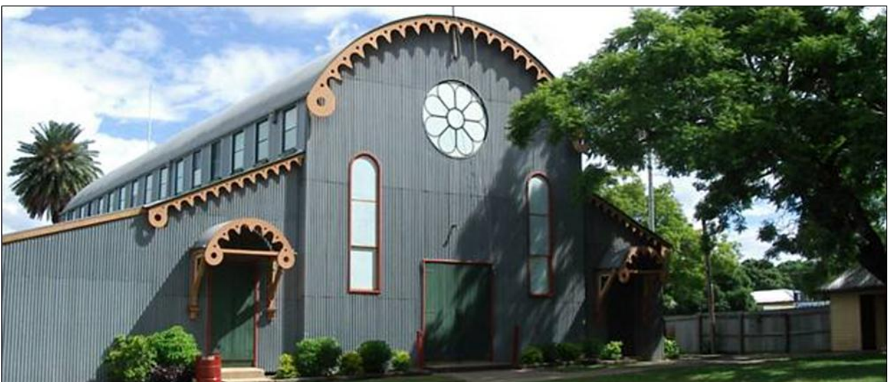
Plate 19: CZB08, north-west elevation of CZB T.J. Ford Pavilion, Showground Complex: Corner of Villiers and Dobie Streets, Grafton (Source: Biosis 2012).
