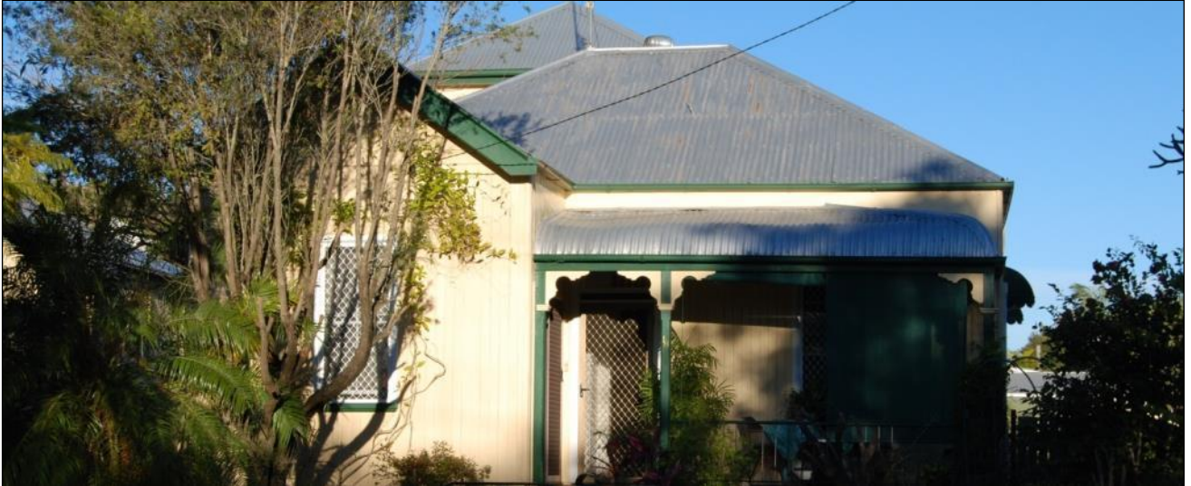
Plate 26: CZB25, north-west facing elevation of 18 Kent Street, Grafton
