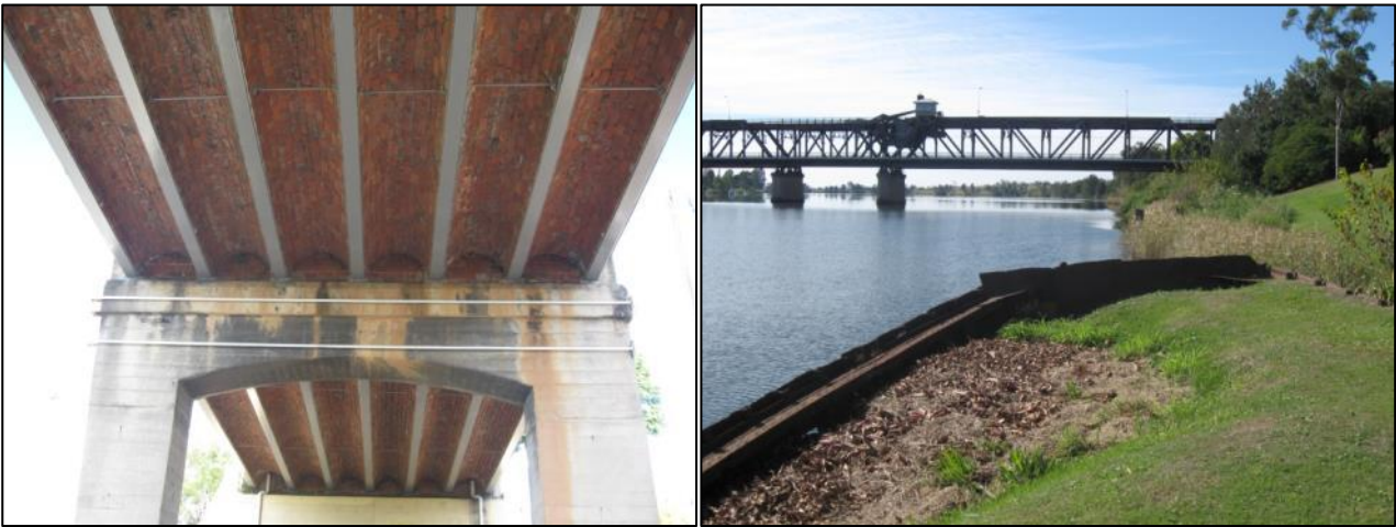
Plate 36: CZB36, detailed brickwork on underside of viaduct exiting Grafton bridge (CZB36) on northern bank (left) and (right), view east from Hull of SS Induna (Source Biosis 2012).
