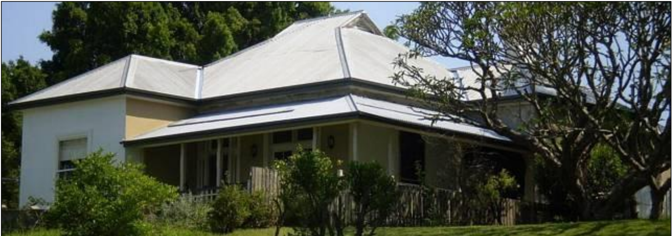
Plate 40: FMW03, 5 Fitzroy Street seen from the Riverbank (Source: Clarence Valley Council).
