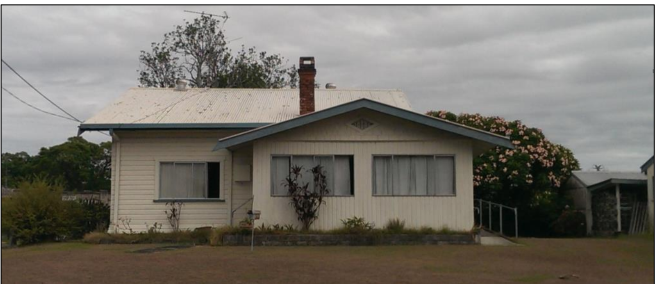
Plate 28: CZB31, south-west facing elevation of 7 Greaves Street, Grafton (new heritage item)
