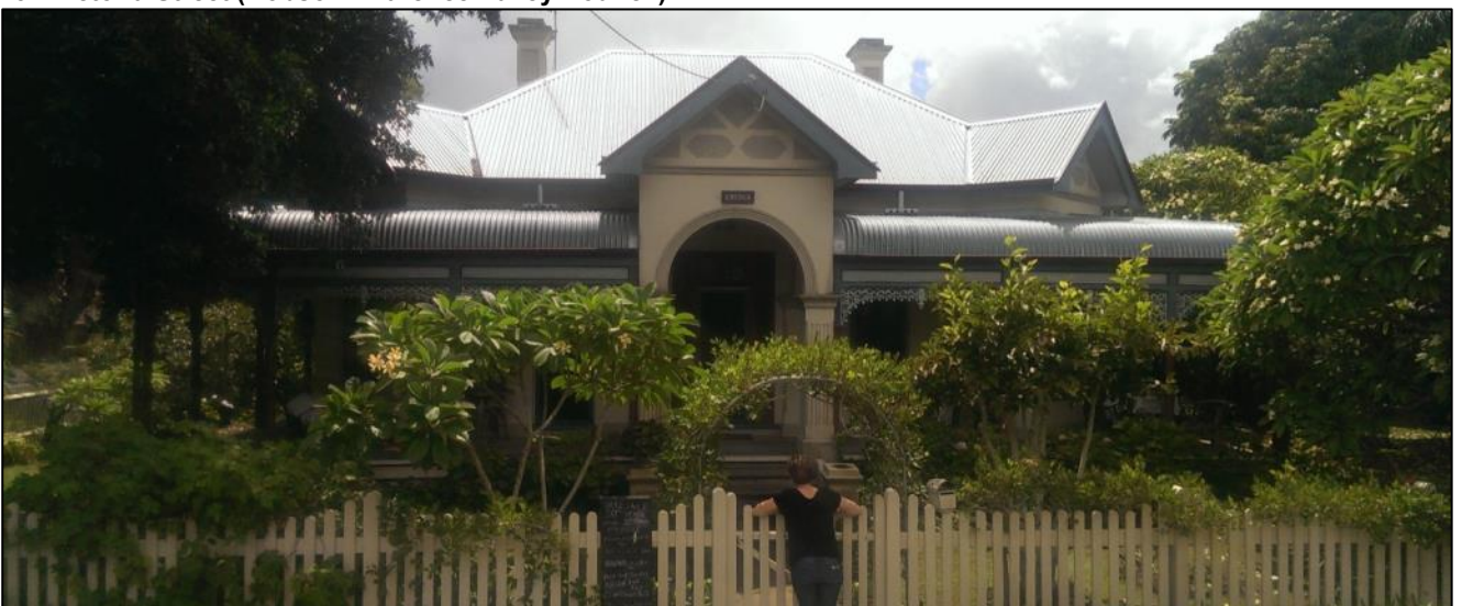
Plate 47: FMW24, north facing elevation of Arcola (Source: Bosis 2014)
