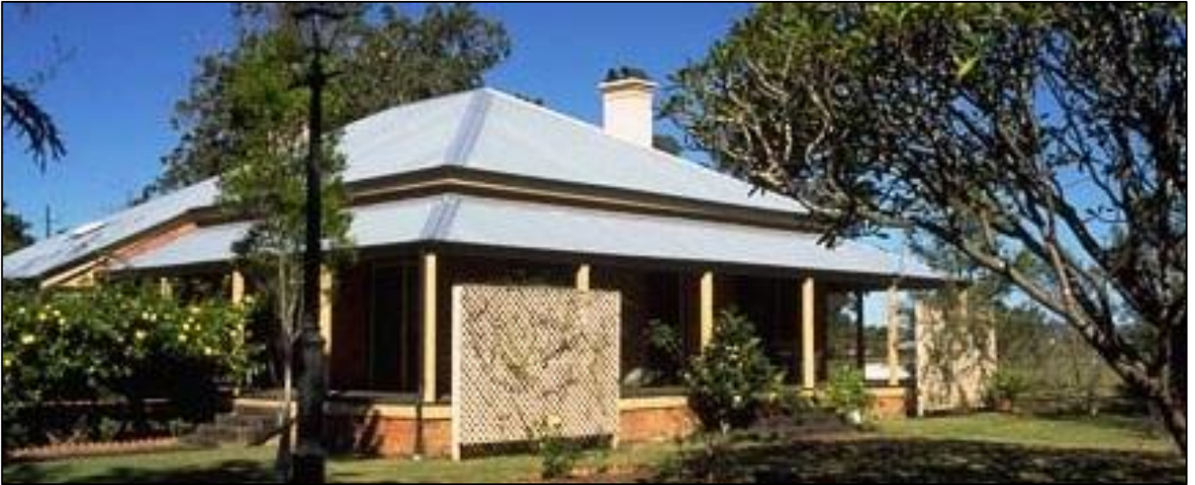
Plate 42: FMW13, south-east elevation of The Deanery (Source: Clarence Valley Council)
