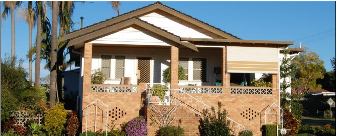
Plate 27: CZB28, north-west facing elevation of 12 Kent Street, Grafton
