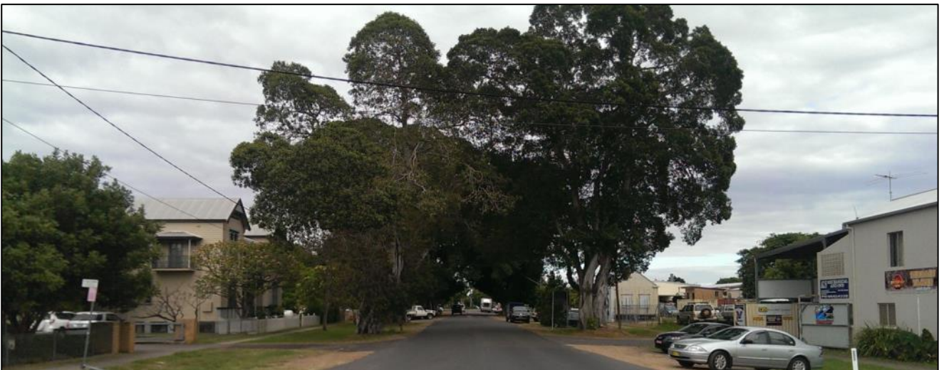
Plate 22: CZB13, North-west facing photograph of Pound Street streetscape between Villiers and Clarence Street. View shows the street trees at this intersection which together with prominent heritage items 'Ravensford' (CZB10) (out of view) and Dunvegan, (CZB11) (visible on the right) forms a significant streetscape within the project area.
