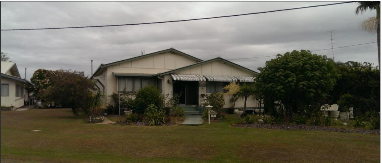
Plate 30: CZB33, south-west facing elevation of 1 Greaves Street, Grafton (new heritage item)
