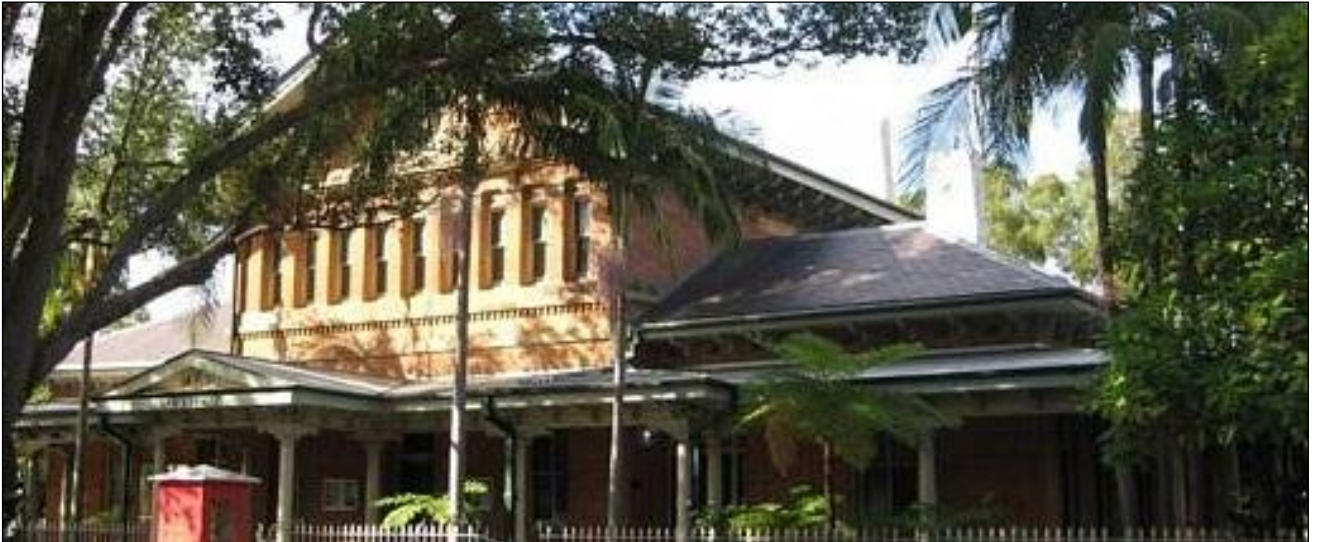
Plate 43: north facing elevation of Grafton Courthouse from Victoria Street (Source: Clarence Valley Council).
