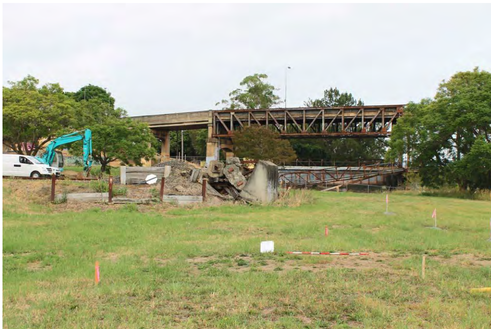
Figure 10: Test Trench 1 looking west prior to excavation.
