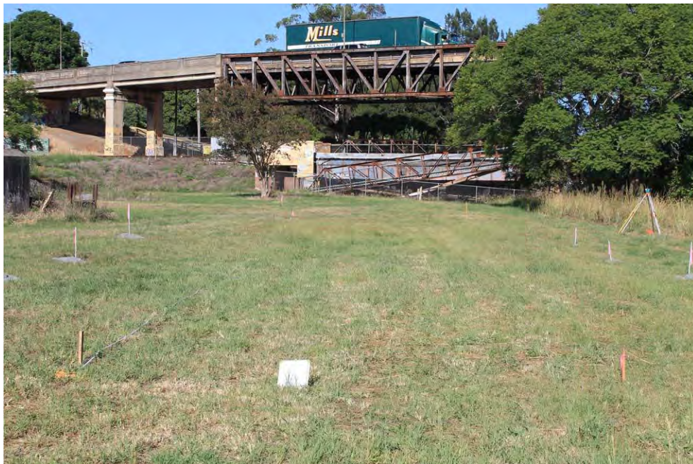
Figure 14: Test Trench 2 before excavation looking west.
