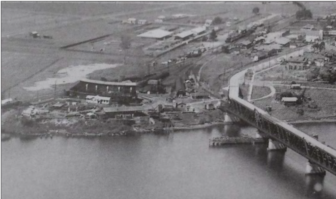
Figure 4: An aerial view of the Clarence River Bridge after construction in the 1930's. Many now-demolished elements of the Railway Terminus area (PB36 and PB37) occupy a large area east of the bridge.
