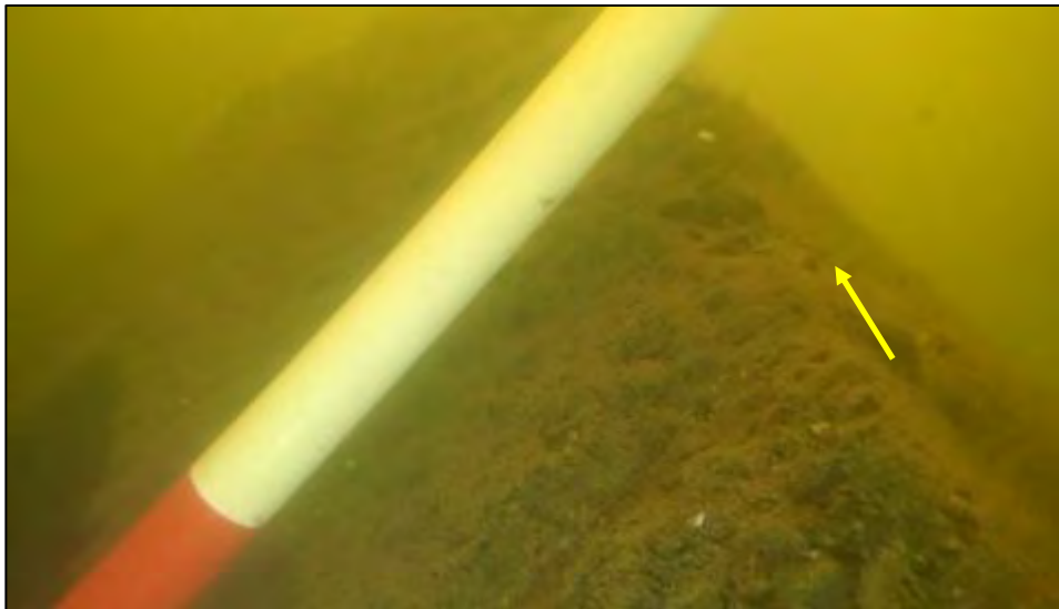
Photograph 12: Concrete pillar sleeve with corrugated at remote sensing feature 2 (yellow arrow)
