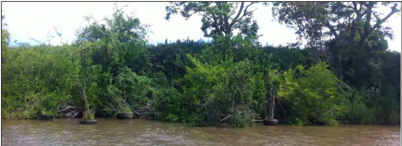
Photograph 10: Derelict wharf from aboard Delta Tauril . (Photo: Mapping & Hydrographic Surveys)
