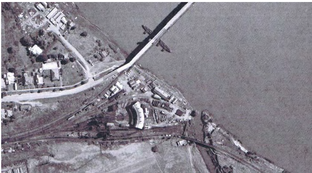
Figure 6: Aerial Image of the South Grafton Locomotive Depot – note the works depot on the bank of the Clarence River
