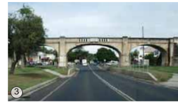
Plate 2.19: Railway bridge over local road, Grafton.
