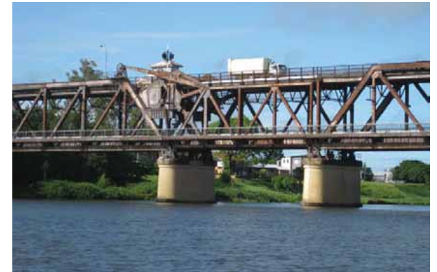
Plate 2.14: Double deck bascule span
