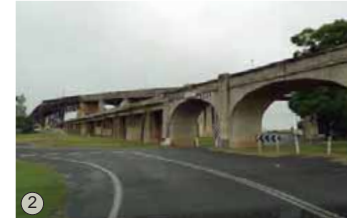
Plate 2.18: Railway viaduct, Grafton with road viaduct & Grafton Bridge beyond.
