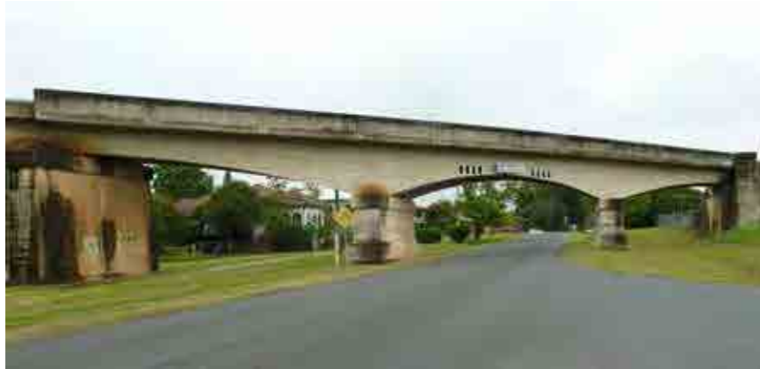
Plate 6.4: Existing railway viaduct over Pound Street, Grafton
