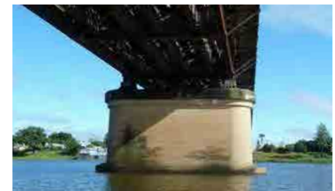
Plate 6.9: Slightly tapering pier shape with rounded pier ends on the existing Grafton Bridge
