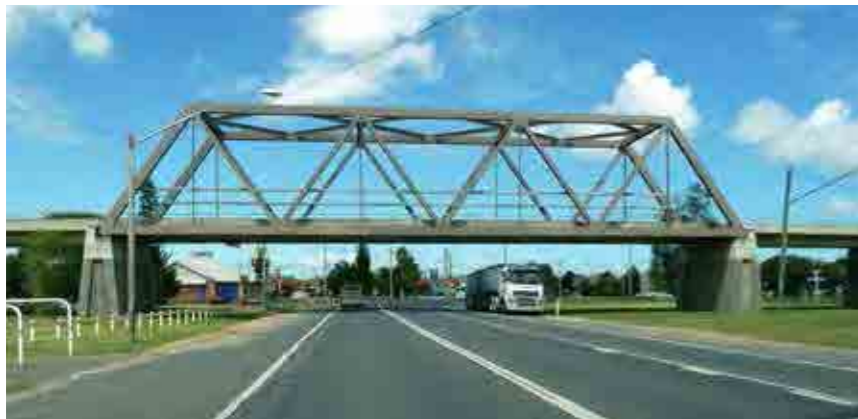
Plate 6.5: Existing railway bridge over the Gwydir Highway, South Grafton
