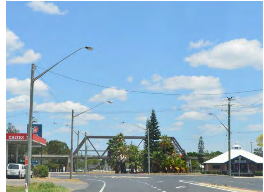
Plate 7.16: View along existing Pacific Highway looking west
