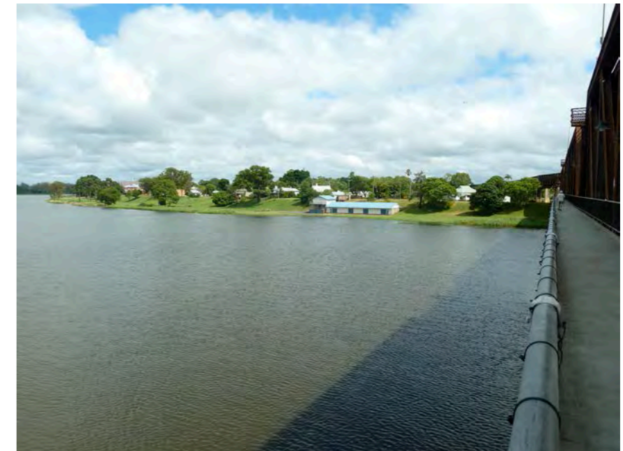
Plate 7.8: Pedestrian path on the downstream side of the existing bridge, looking south
