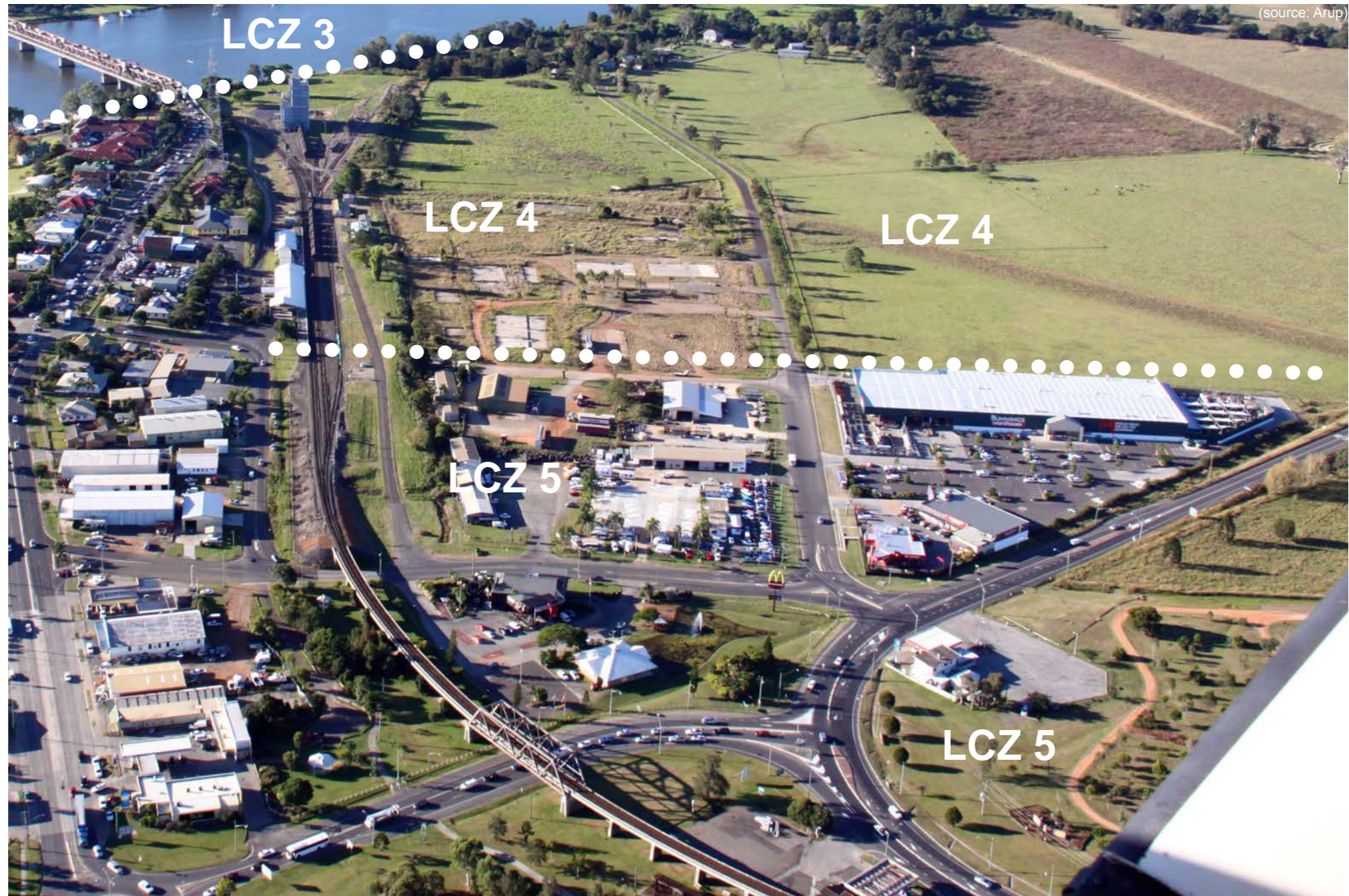
Plate 7.21: Existing landscape character of the South Grafton area without the proposed bridge and approach roads
