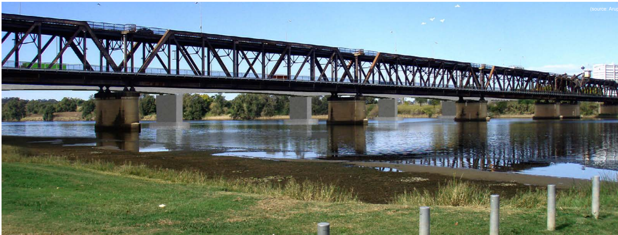
Plate 7.24: Before and after artist impressions of Viewpoint 5. Artist impression represents anticipated view during opening year.
