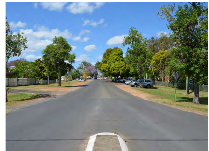
Plate 7.3: View along existing Clarence Street looking south west
