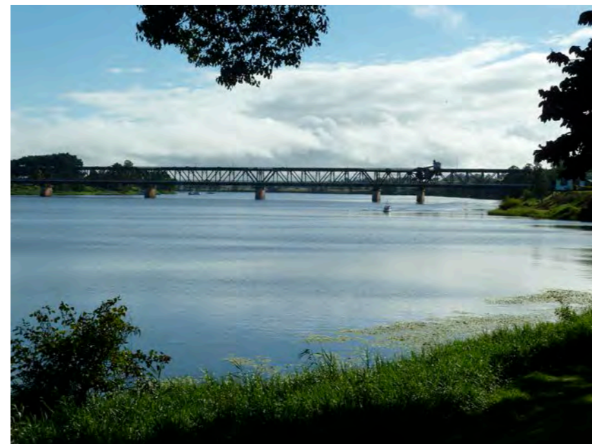
Plate 7.7: The existing bridge viewed downstream from South Grafton CBD
