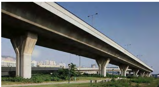
Concrete box-girder bridge – Kwun Tong, Hong Kong
