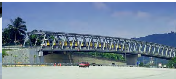
Steel truss bridge – STAR Light Rapid Transit, Kuala Lumpur
