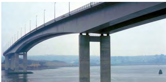
Steel plate girder bridge- Foyle Bridge, Derry – Northern Ireland
