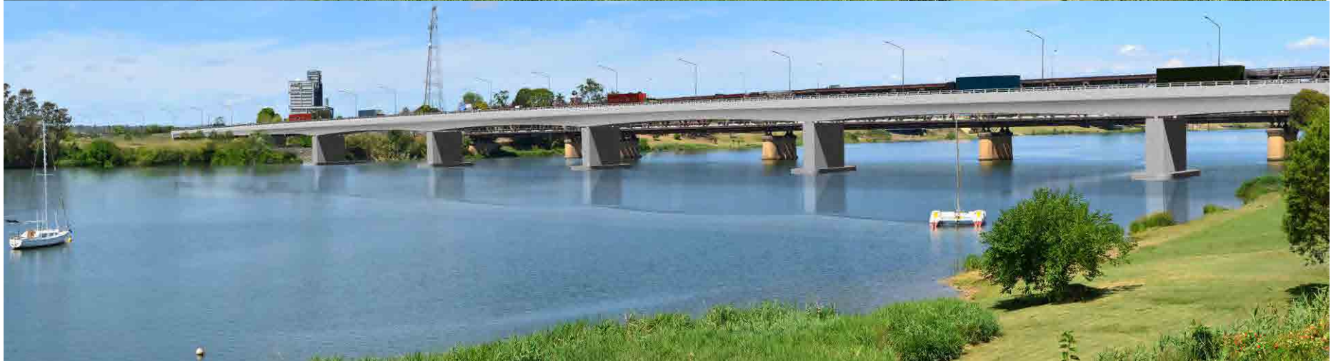
Figure 8-35 Viewpoint 6: Foreground view of the existing bridge and the Clarence River
