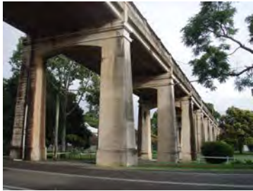
Road viaduct, Grafton.
