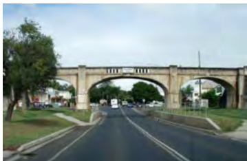
Railway bridge over local road, Grafton.
