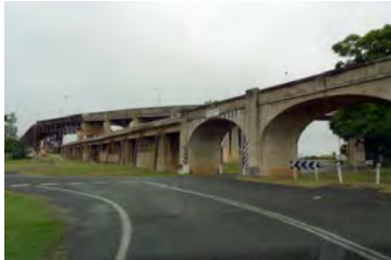
Railway viaduct, Grafton with road viaduct & Grafton Bridge beyond.
