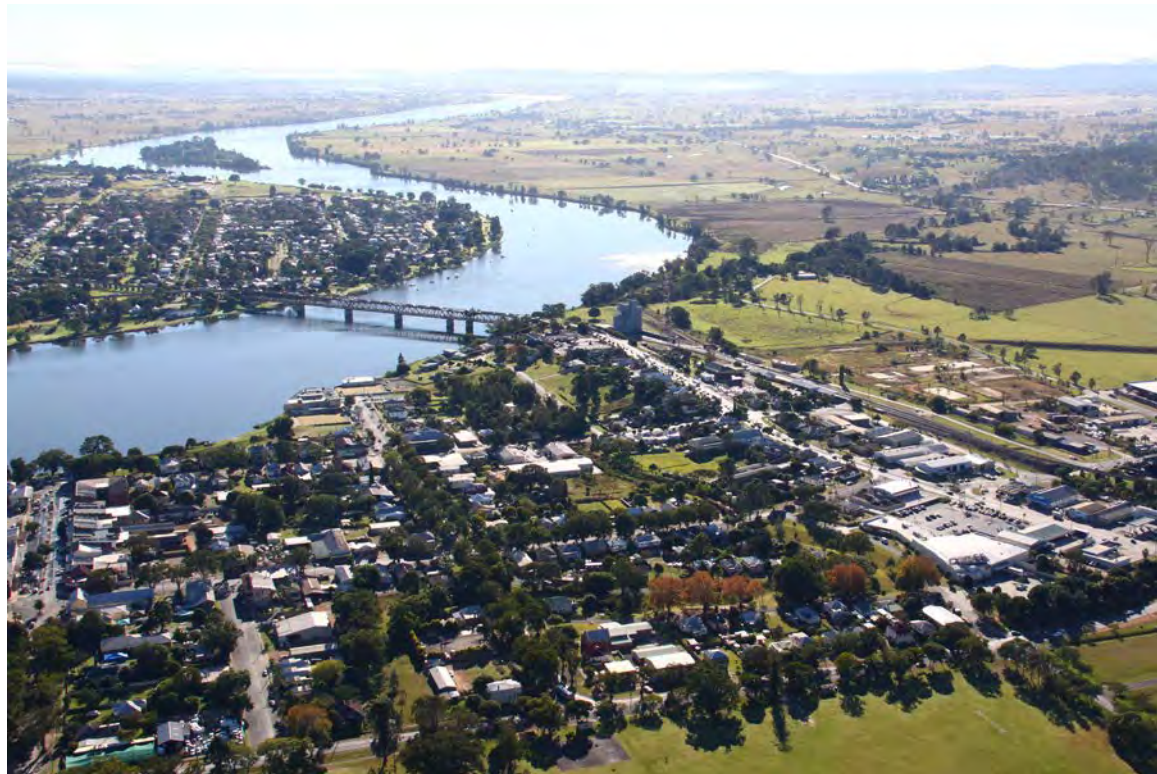
Above: Aerial photograph showing South Grafton's town centre to the west of Bent Street. The light industrial area and agricultural floodplain east of Bent Street is in the background. (Source: Arup 2010)
