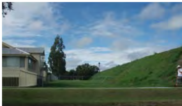
Railway embankment, Grafton.
