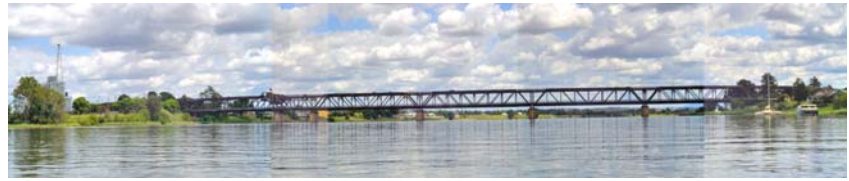
Illustration 13 – view from Clarence River opposite Pound Street Jetty
