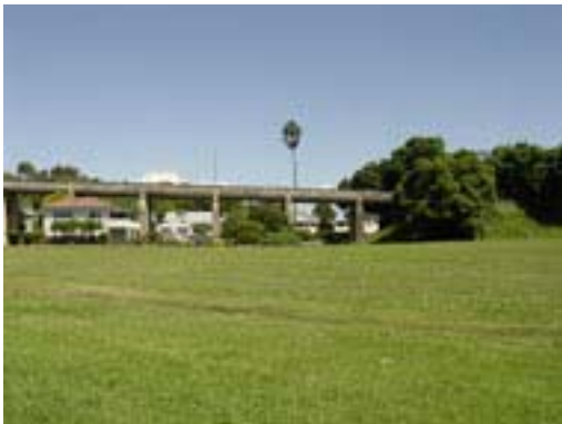
Illustration 25 – side view of the planted embankment
