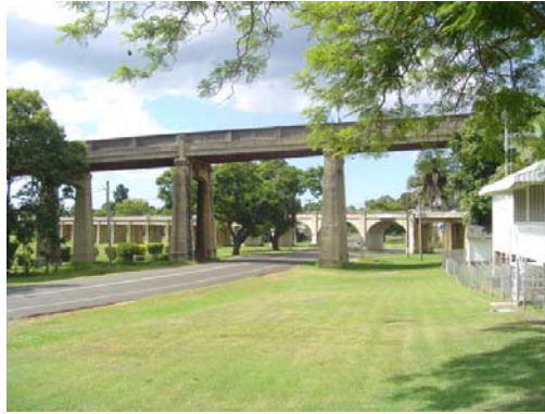
Illustration 4 – northern approach to the bridge
