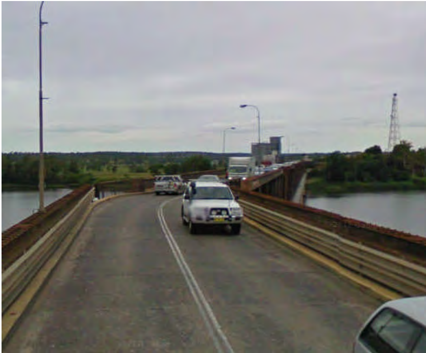
Figure 7: Grafton Bridge 'kinks'
