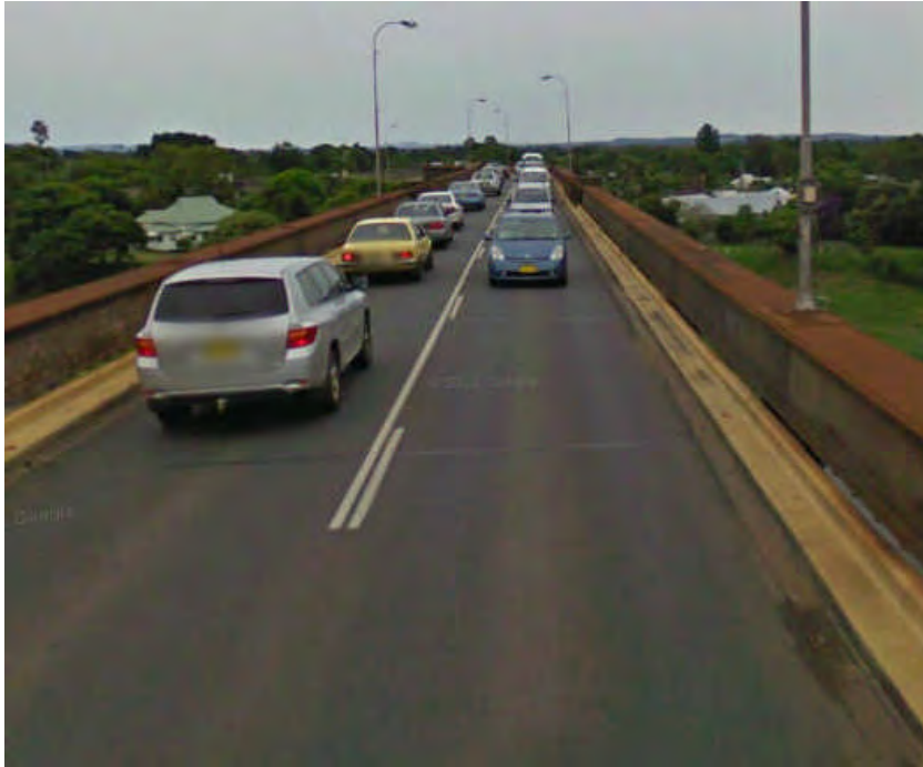
Figure 5: Summerland Way – lane configuration and capacity
