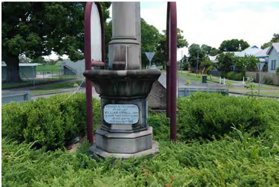
Plate 4: William Small Memorial, Intersection of Ryan Street (Gwydir Highway) and Skinner Street, South Grafton.
