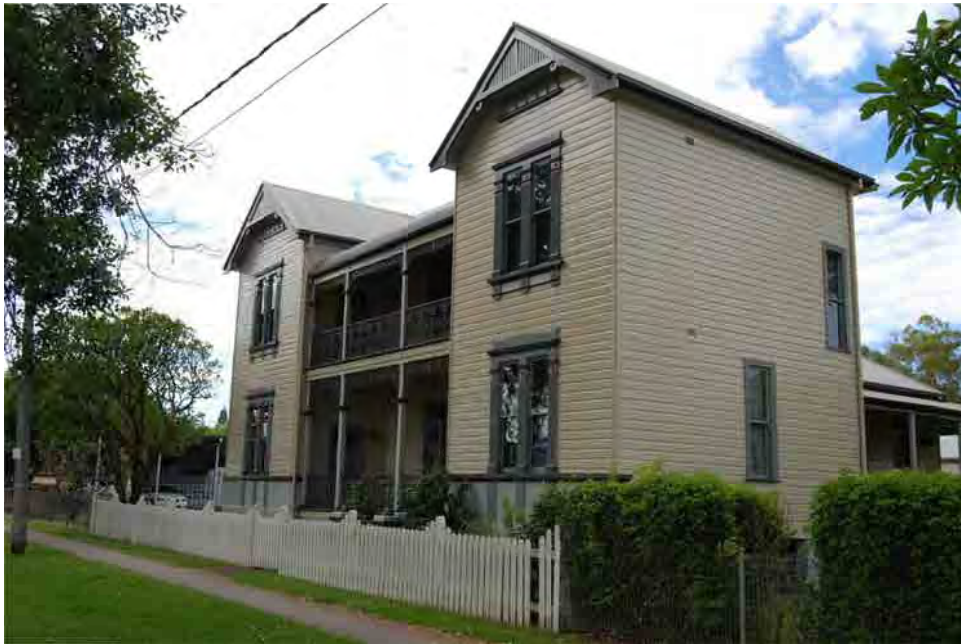
Plate 11: “Dunvegan”, TAFE and grounds in Pound Street, Grafton, listed on the LEP and REP, and the location of a potential archaeological site.
