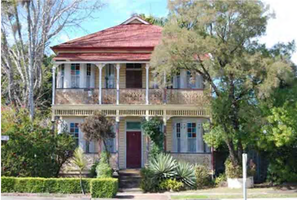
Plate 34: “Ravensford”, 36 Villiers Street. Also potentially impacted by Options E and A.
