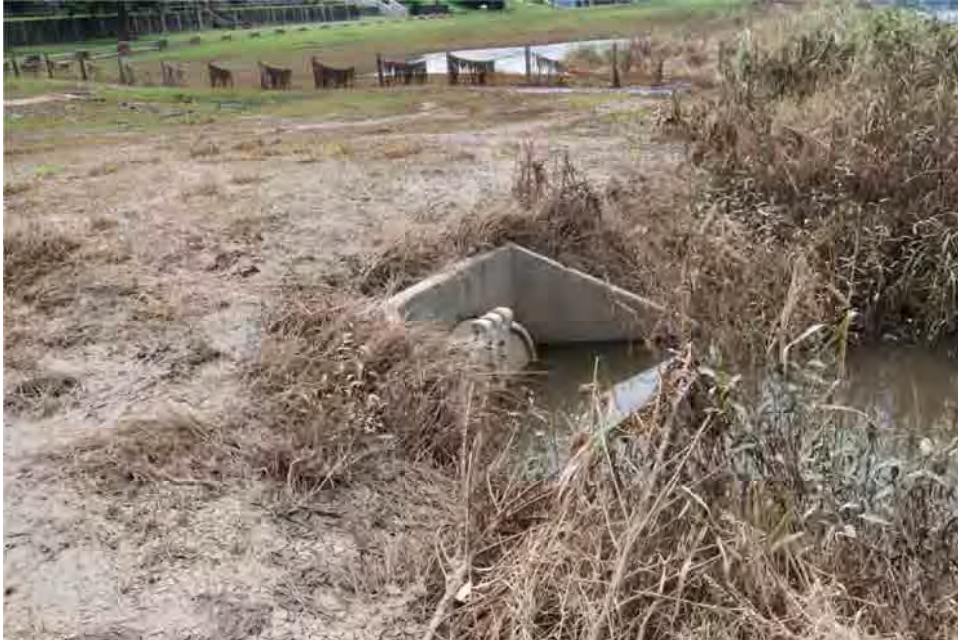
Plate 10: Drain outlet at site of punt ramp on Villiers Street.
