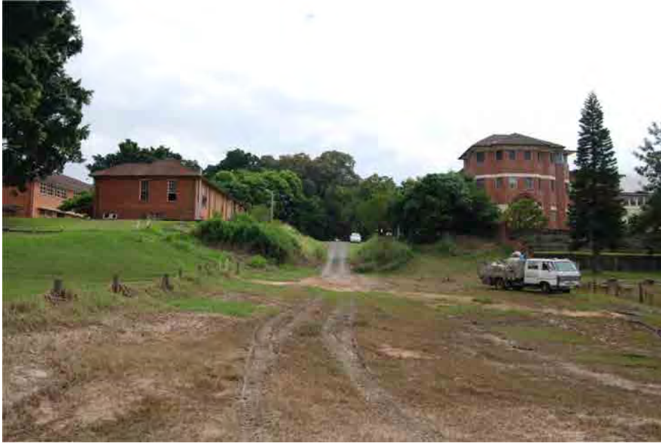
Plate 9: View from site of punt ramp towards Villiers Street, where Option E connects on Grafton Side.
