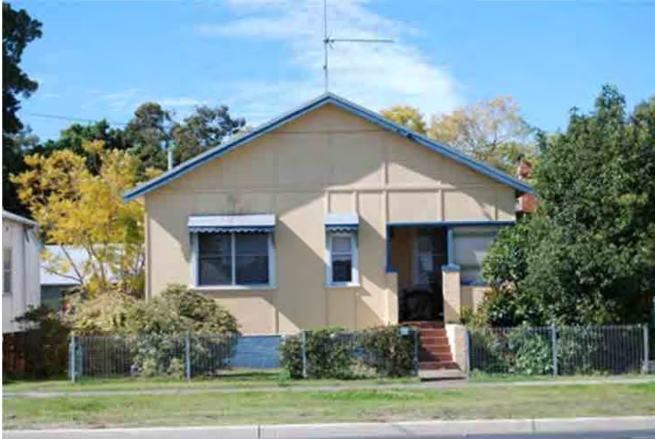
Plate 20: 16 Villiers Street, between Fitzroy and Pound Streets. Listed on the CVLEP 2011.
