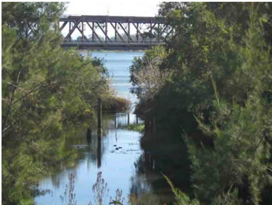
Plate 35: Alipou Creek, view of Grafton Bridge and wharf relics.
