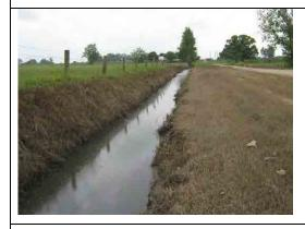
Plate 19. Degraded stormwater drain along North Street – Options 14 and 15
