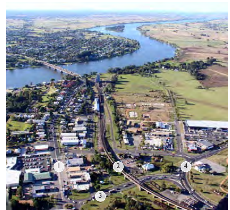
Above: Road and rail approaches to Grafton Bridge at South Grafton (1) Bent Street, (2) North Coast railway, (3) Gwydir Highway, (4) Pacific Highway
