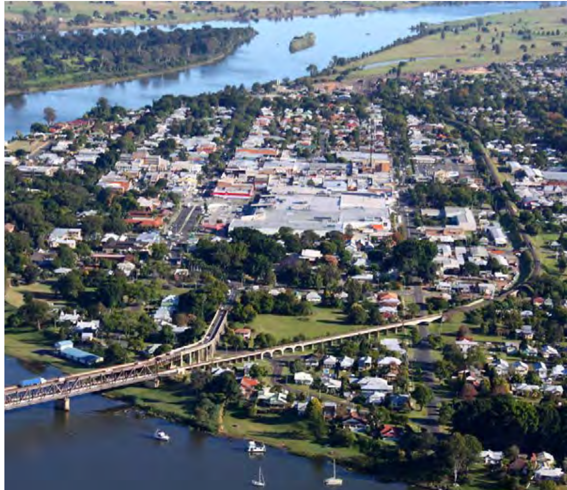
Left: Relationship of the existing approach road viaduct and railway viaduct to the local street grid in Grafton (Source: Arup 2010).
