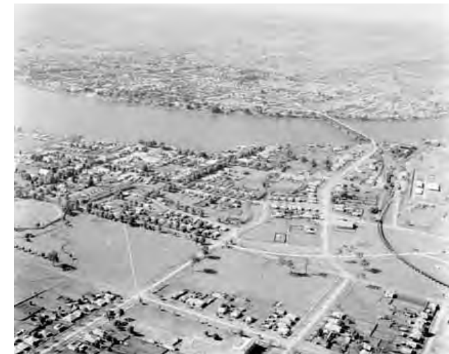
Top: View of Grafton Bridge with the bascule span open. (Source: Clarence Valley Council 2007, A thematic History of the City of Grafton )
