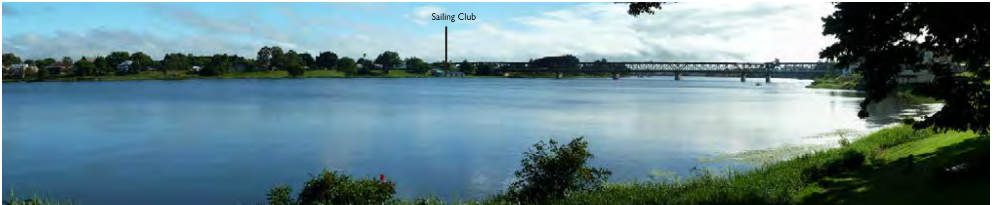
View from upstream of the Grafton Bridge where Option A alignment would cross the Clarence River
