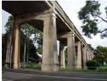
Road viaduct, Grafton.
