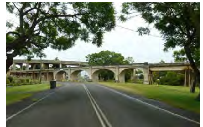
View of the existing viaduct network in Grafton
