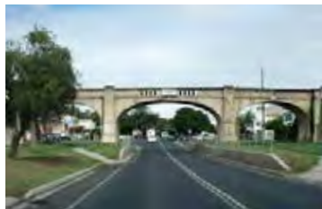
Railway bridge over local road, Grafton.
