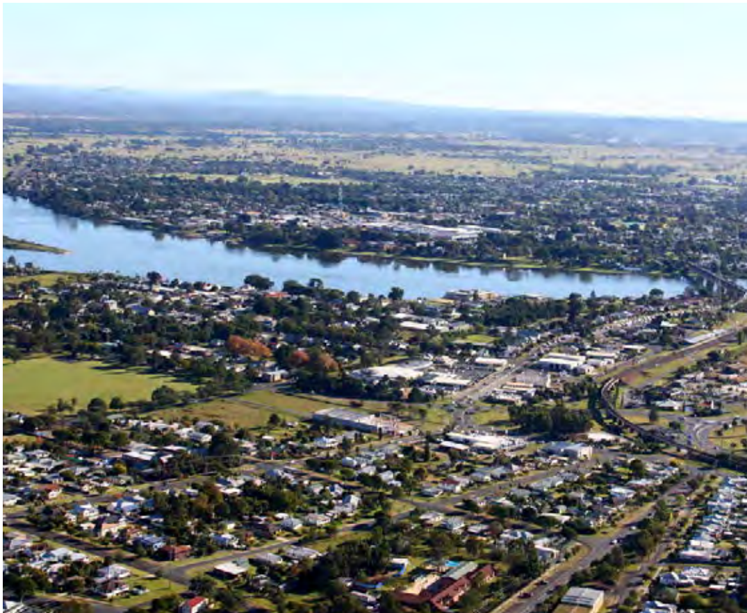
Aerial view from South Grafton across the Clarence River to Grafton (Source: Arup 2010).
