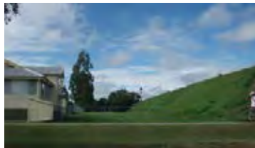
Railway embankment, Grafton.
