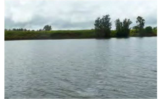
View of proposed bridge abutment location on the South Grafton foreshore
