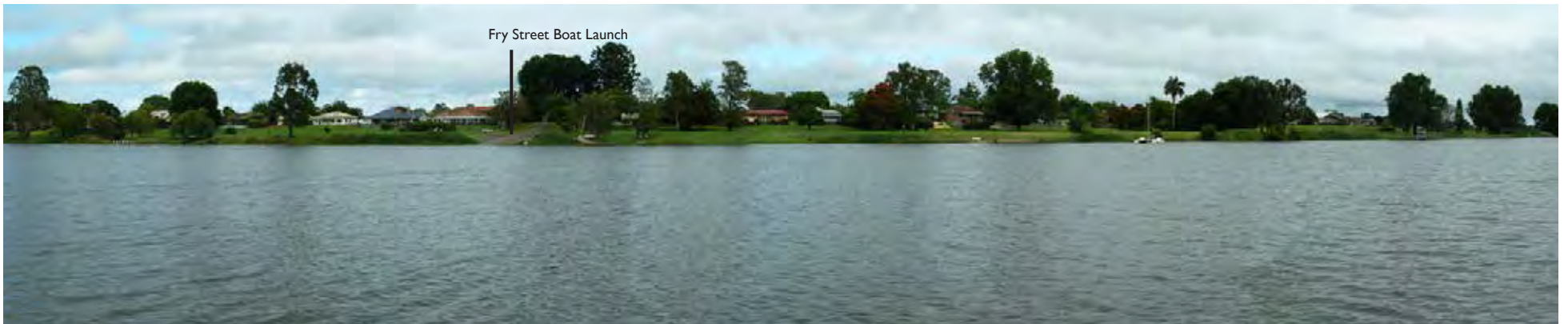
View of the Grafton foreshore and bridge abutment location for the Option 11 alignment crossing of the Clarence River
