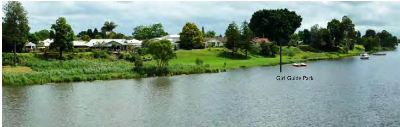
View of Grafton foreshore amenity where Option C alignment and abutment would be located
