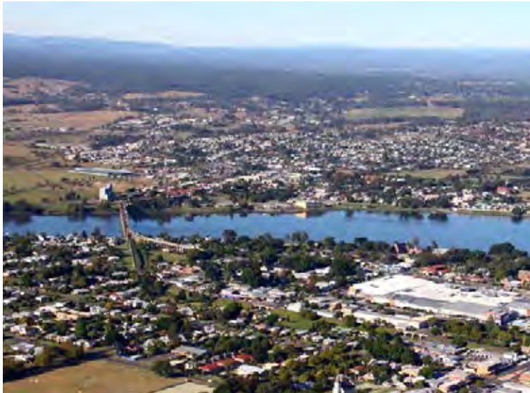
Aerial view from Grafton, across the Clarence River to South Grafton (source: Arup 2010).
