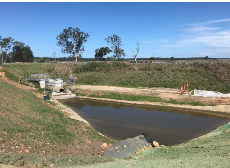
Figure 9 Grass strike from hydroseeding and polymer controls on batters surrounding clean water basin at Fill 2
