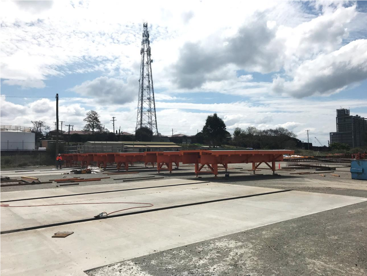
Figure 5 Mould segments in the process of construction onsite
