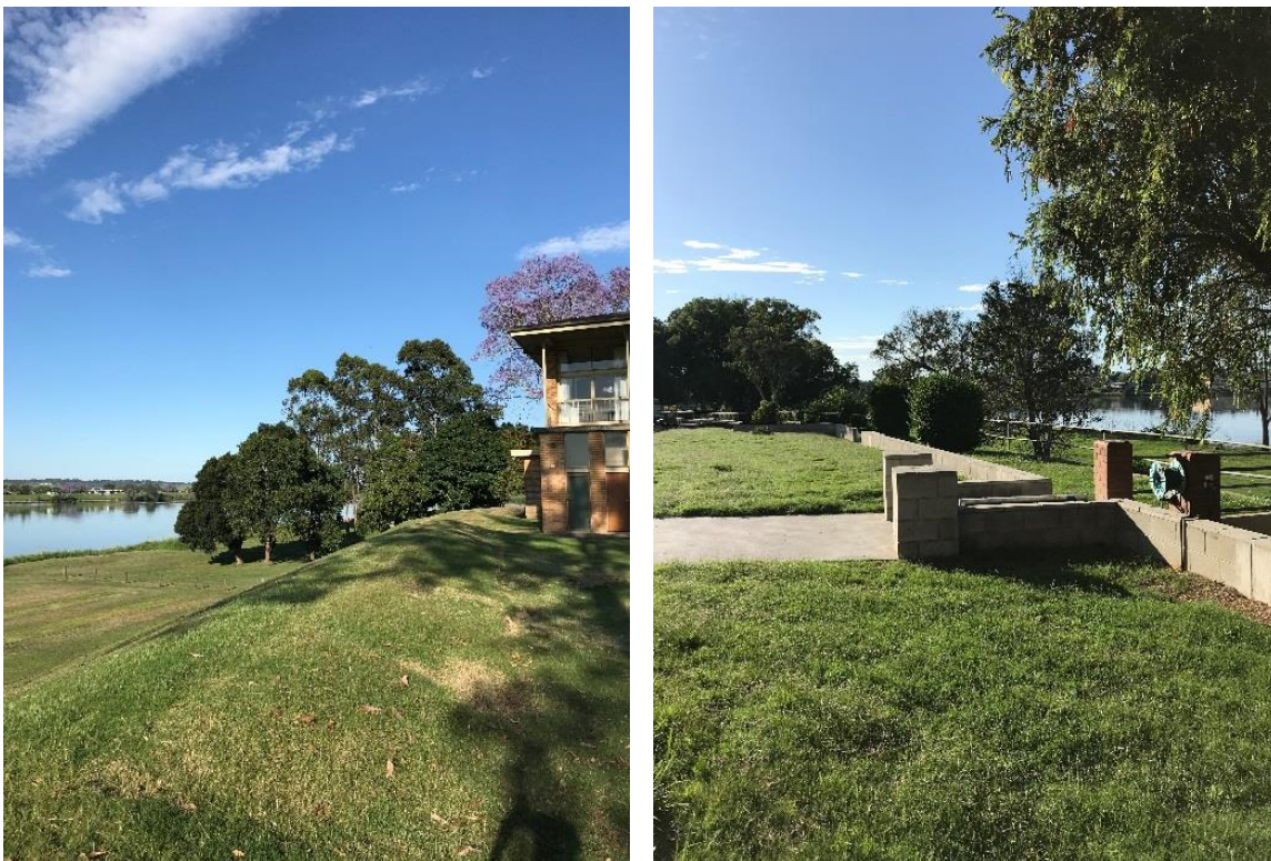
Figure 1 Completed levee works in Grafton at (a) NG04 and (b) LPO111
