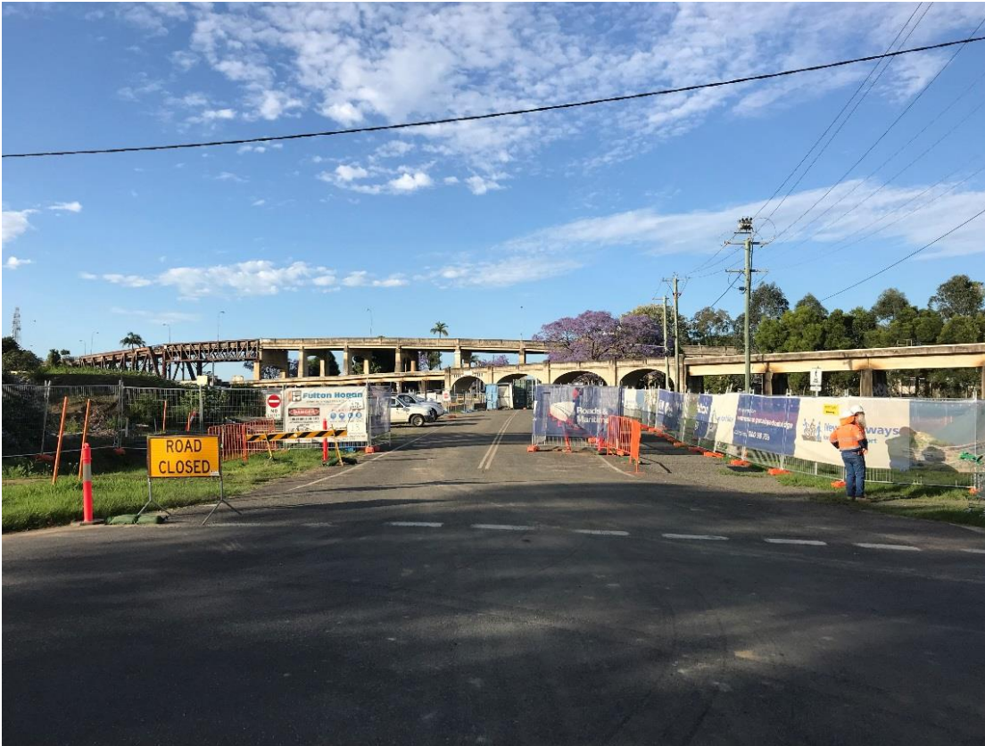
Figure 4 Permanent closure of Kent Street
