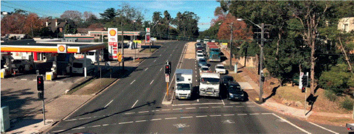
Pacific Highway and Redleaf Avenue, Wahroonga: Three southbound lanes and two northbound lanes with a dedicated right turning lane
