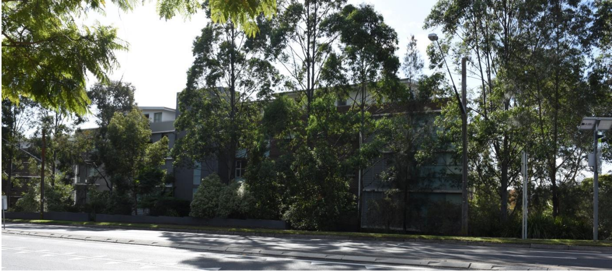
Figure 2-8 View to 1389-1397 Pacific Highway, Warraroo, looking east. High density residential development within the LCZ comprises larger built forms with mature tree and shrub planting within the front yard setbacks
