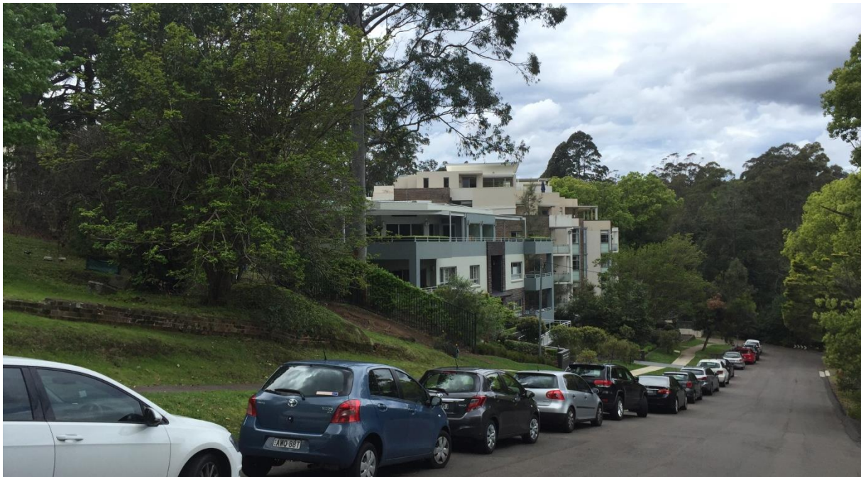
Figure 5-14 Apartments at 16-18 Boyd Street, Turramurra. Photo taken from Boyd Street looking east along the road towards the apartments
