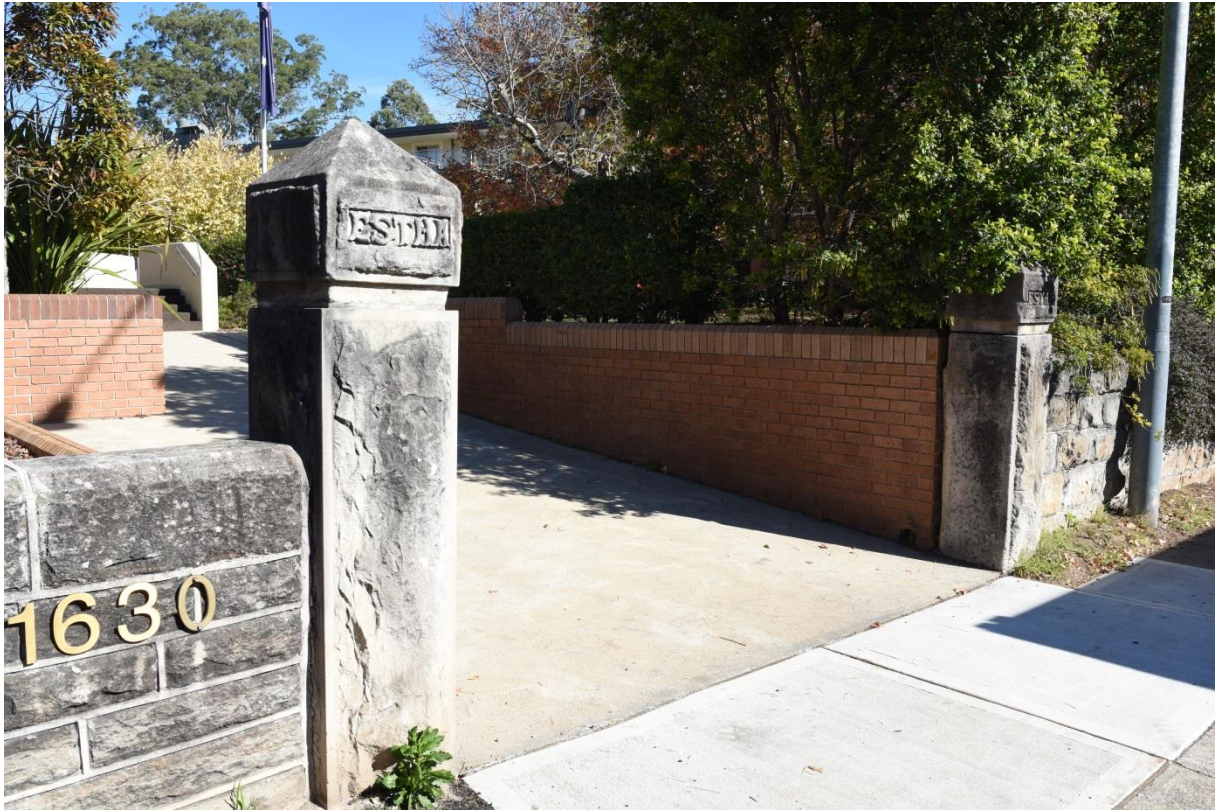
Figure 5-2 Estha Gates (locally listed heritage item) and the existing newer sandstone wall and the entry driveway to the aged care facility
