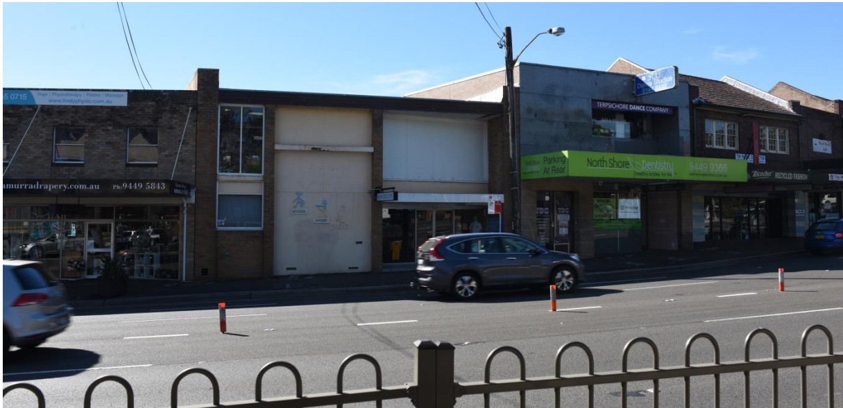
Figure 2-14 The northern verge of the Pacific Highway at the Kissing Point Road intersection at Turramurra (looking north)
