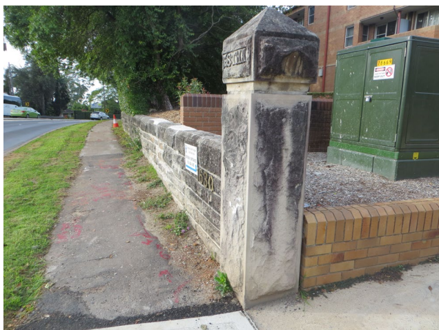
Figure 3-11: Existing retaining wall and planting on the property at 1614-1634 Pacific Highway, Wahroonga, including the 'Estha' gate post in the foreground (looking east from the Pacific Highway on the north western extent of the property)
