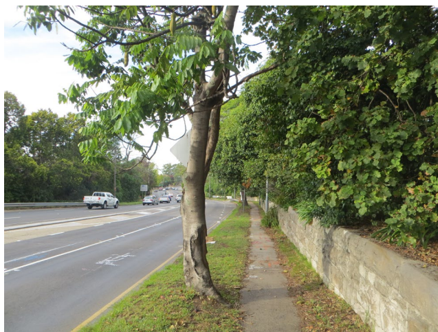
Figure 3-12: Existing retaining wall and planting on the property at 1614-1634 Pacific Highway, Wahroonga, (looking east from the Pacific Highway on the north eastern extent of the property)
