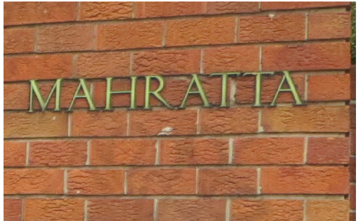
EXISTING RETAINING WALL
