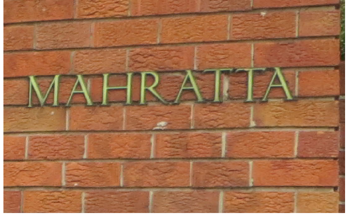
EXISTING RETAINING WALL
