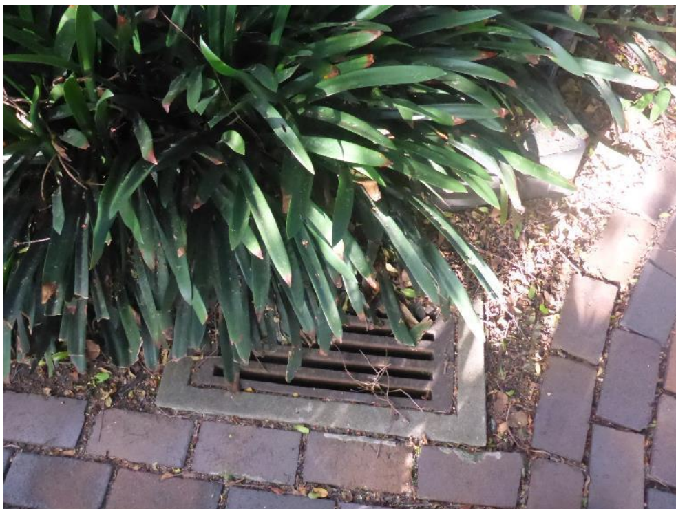
Plate 20 Evidence of sub-surface drainage infrastructure within the Mahratta [12] grounds
