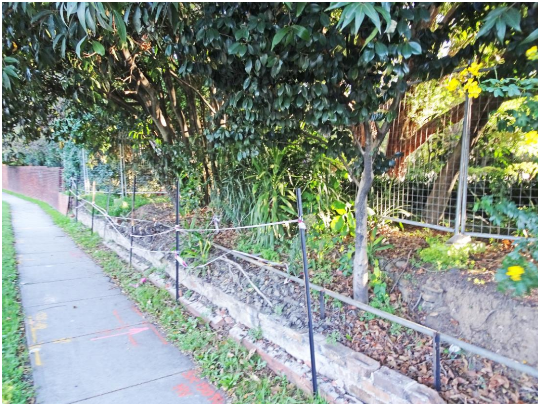
Plate 6 Section of removed wall on the Pacific Highway boundary
