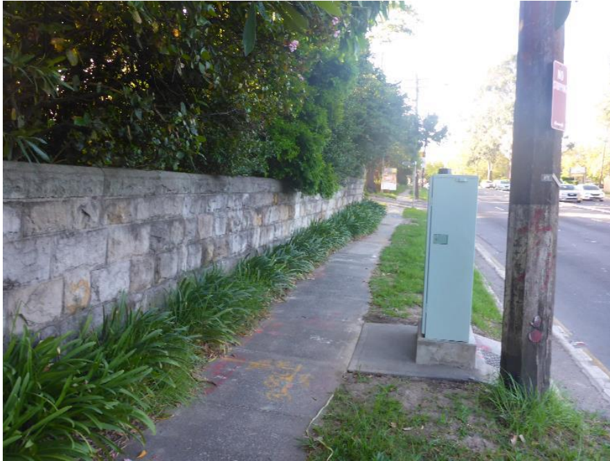
Plate 10 View of stone boundary wall of heritage listed Kyeamba dwelling [17] adjacent to Yaamba [29] and road reserve area with evidence of sub-surface infrastructure works, facing north-west
