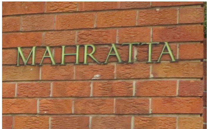
EXISTING RETAINING WALL
