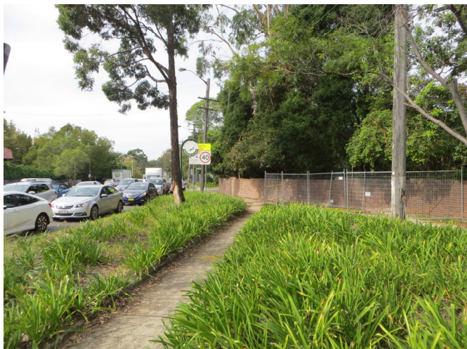
Figure 3-28: Existing brick wall in front of 2 Fox Valley Road, Warrawee (looking south from the intersection of Pacific Highway and Fox Valley Road)
