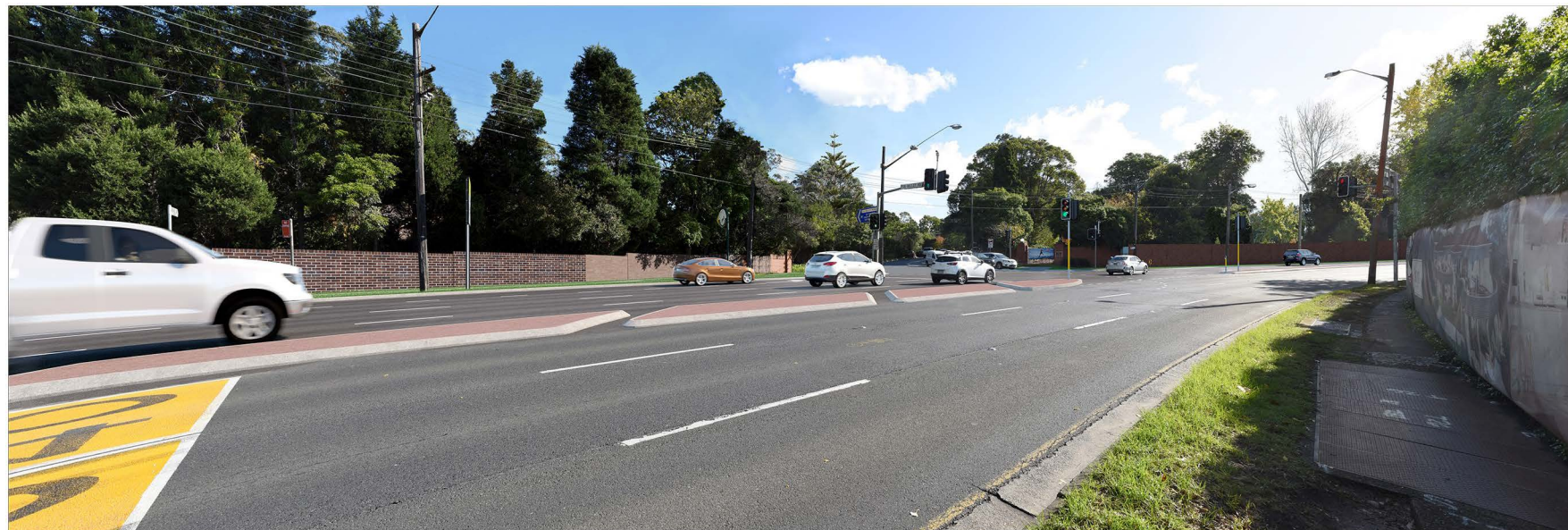
Visualisation of Proposal (Just After Construction) – South of Fox Valley Road on approach to the intersection towards “Mahratta” / School of Practical Philosophy - Wahroonga (looking north west)
