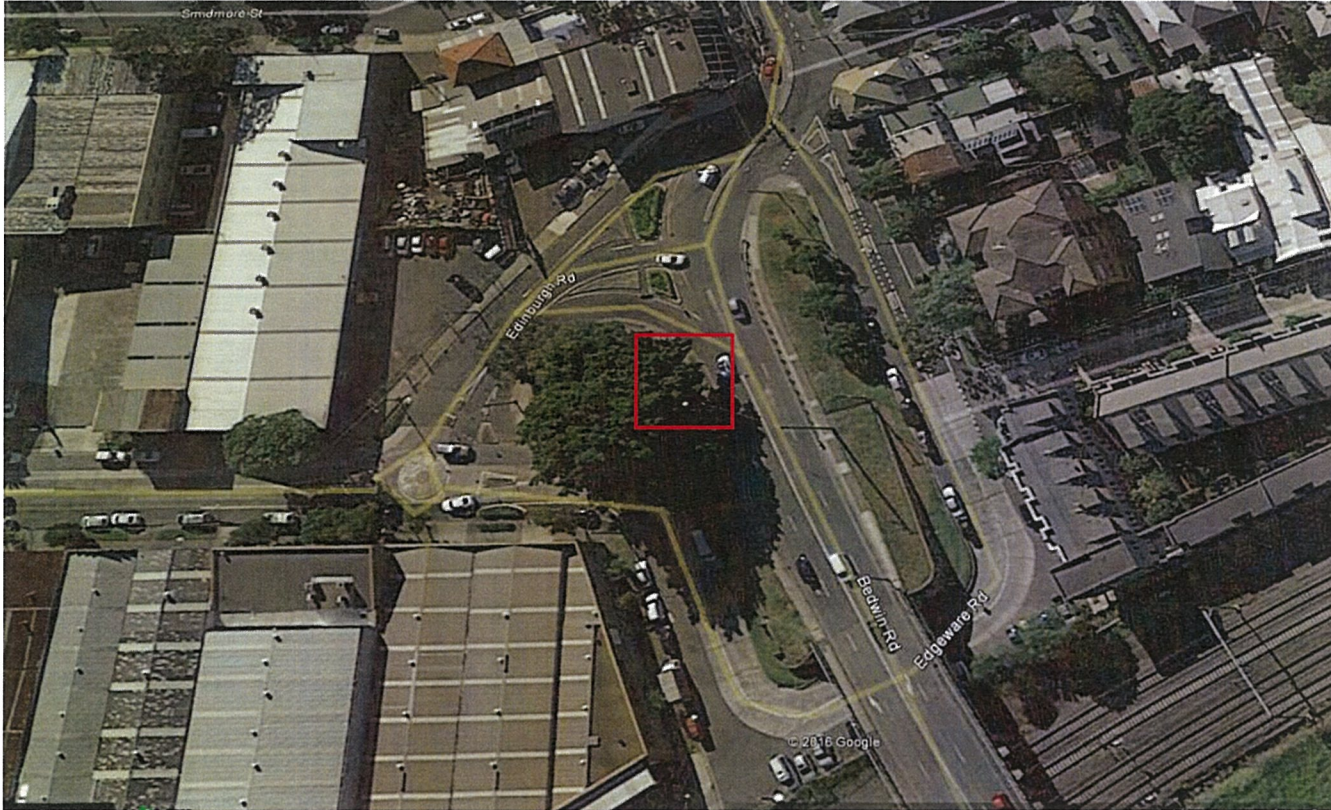
Marrickville Worksite (Bedwin Road)
